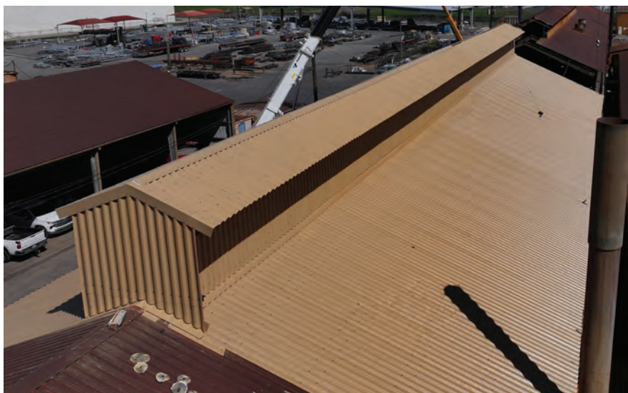
Roof with Enduro Composites panels installed.
