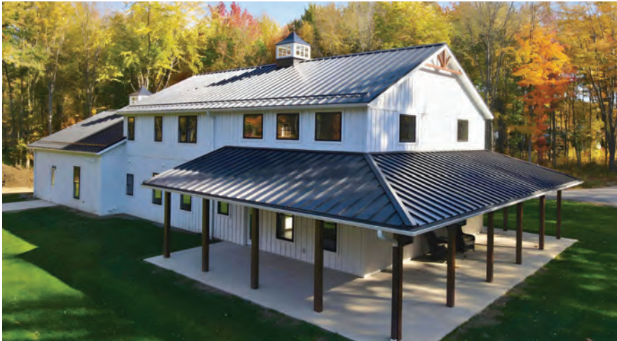
Metal roofing project. COURTESY OF METAL EXTERIORS
