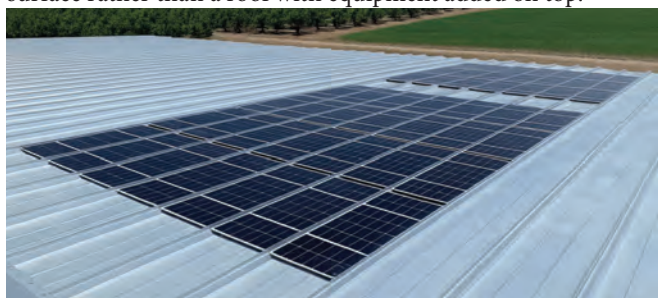
SunSteel™ integrated solar on MBCI Double-Lok™ metal roofing panels. PHOTO COURTESY OF MBCI / CORNERSTONE BUILDING BRANDS.
