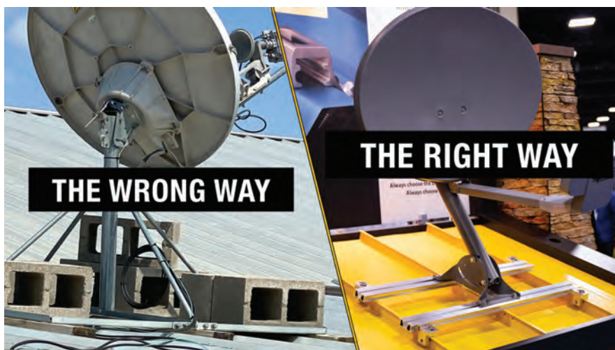
Rooftop mounting systems that allow the free flow of rainwater can reduce the risk of rust.
