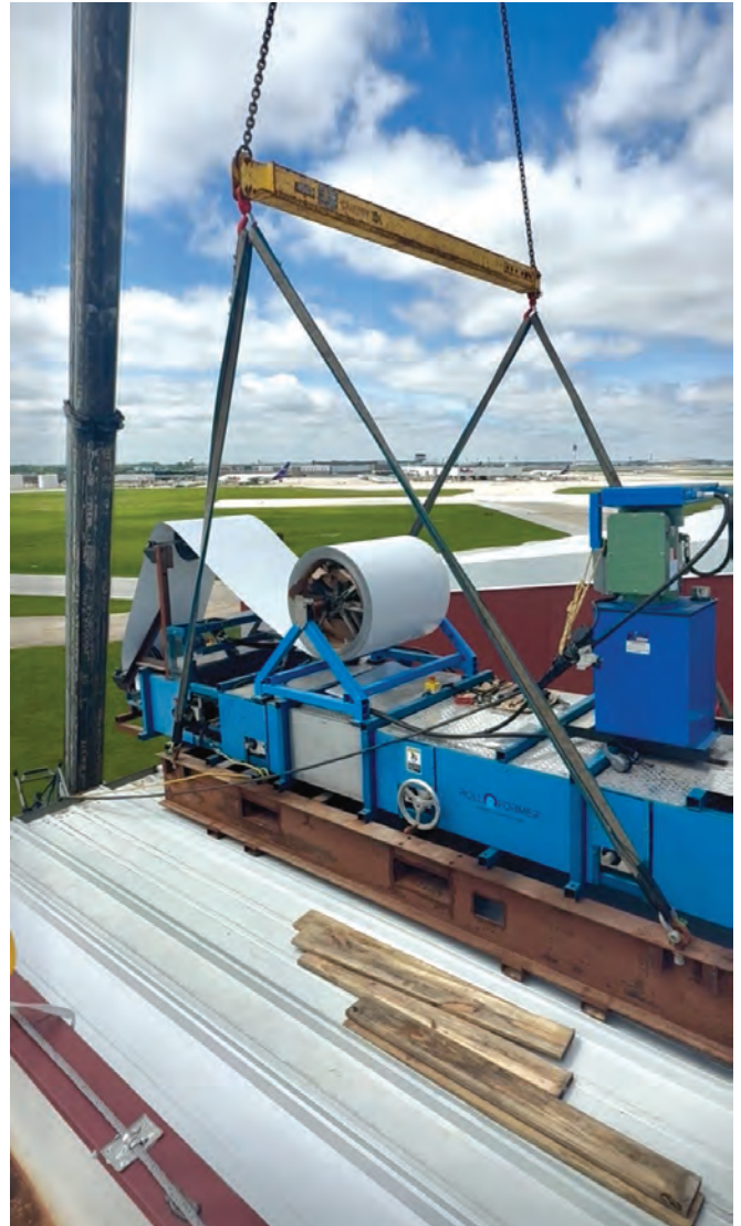
A Roll Former LLC portable machine is hoisted onto the roof to make panels just steps from where they will be installed. PHOTO COURTESY OF INDIANA METAL.
