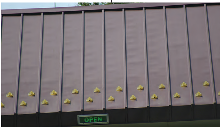
Vantage point and time of day can greatly influence the appearance of oil canning on a metal roof. The bottom photo was taken at approximately 11:15 a.m. on a sunny day. The top photo was taken approximately one hour later under more direct sunlight from a point about 10 feet to the right. The oil canning is easier to spot in the top photo.
