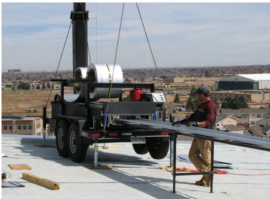
A New Tech roll former cranks out standing seam panels on the roof deck. PHOTO COURTESY OF NEW TECH MACHINERY.
