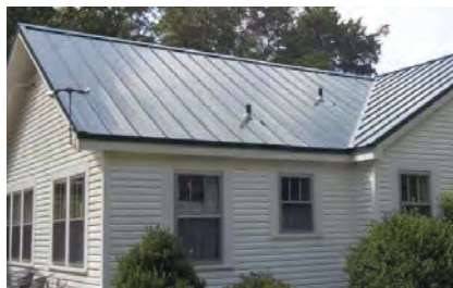
MasterCraft Metals in Tucson, Ariz., forms three fluted striations into its standing seam panels (top) to minimize the appearance of oil canning. Sunshine Metal Works of Oxford, Ala., uses ribs or striations in its panels (below).
