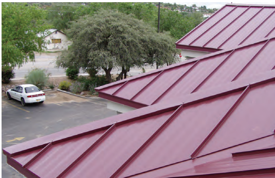
MasterCraft Metals in Tucson, Ariz., forms three fluted striations into its standing seam panels (top) to minimize the appearance of oil canning. Sunshine Metal Works of Oxford, Ala., uses ribs or striations in its panels (below).
