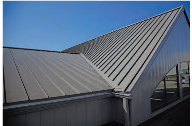
Hangers should be no more than 24 inches apart to ensure the gutters stay in place. PHOTO COURTESY OF FIRESTONE
