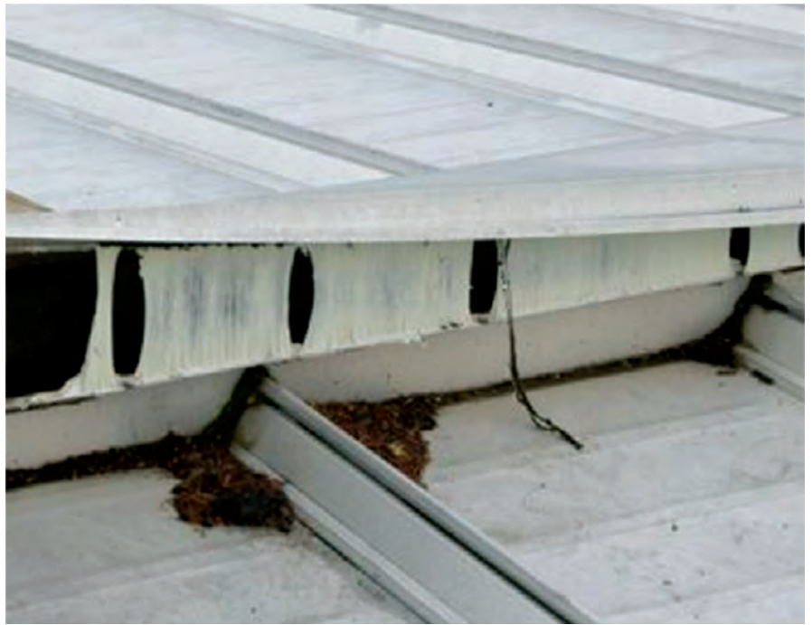
Figure 6: Webbing and cohesion of a proven formulation after 35 years of service. PHOTO COURTESY OF ROB HADDOCK, METAL ROOF ADVISORY GROUP, LTD
