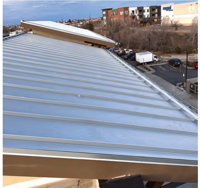
Although the region received only a moderate 57" of snow each year, On Point Contracting solved the snow avalanching problem at the WoodSpring® Suites Hotel in Littleton, Colorado, by installing a snow retention system designed by Rocky Mountain Snow Guards. PHOTO COURTESY OF ROCKY MOUNTAIN SNOW GUARDS.
