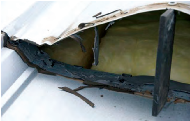
Figure 2: A "Brand X" butyl sealant failure at 5-7 years' service. PHOTO COURTESY OF ROB HADDOCK, METAL ROOF ADVISORY GROUP, LTD
