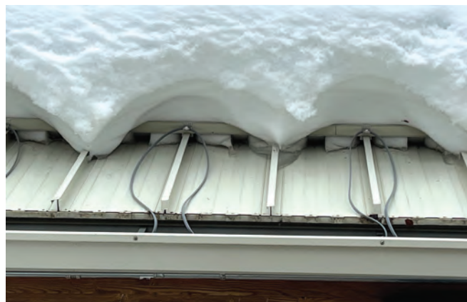
A heated cable system assists with roof and gutter de-icing. PHOTO COURTESY OF FLOTRACE
