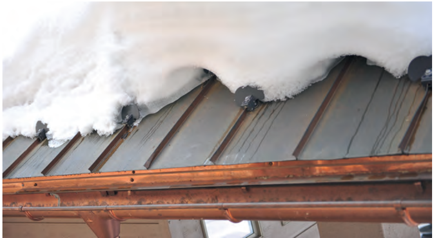
Combining snow guards and a heated cable system provides an efficient snow and ice management system on metal roofs. PHOTO COURTESY OF FLOTRACE
