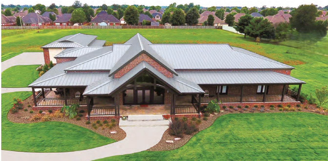
Galvalume roofing delivers exceptional corrosion resistance, especially with an SMP coating. PHOTO COURTESY OF CENTRAL STATES MANUFACTURING
