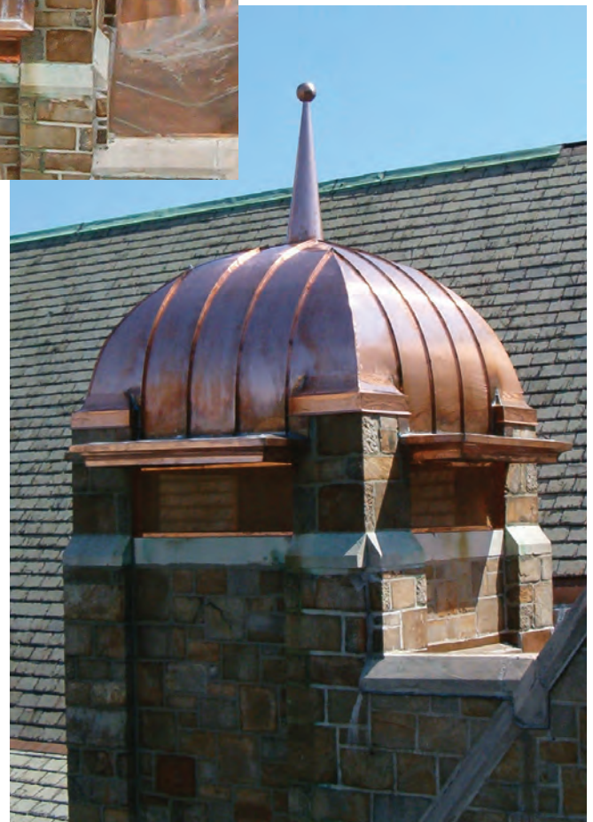
Crocker Architectural of Oxford, Massachusetts, uses a hand seamer for specialty jobs — like this cupola on the First Unitarian Church in Newton, Massachusetts. CROCKER ARCHITECTURAL PHOTOS
