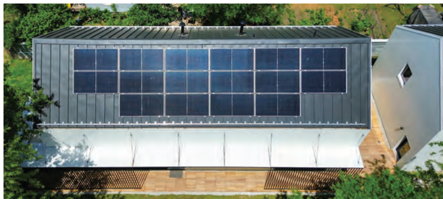
Designed and built by students in the University of Kansas School of Architecture & Design's Studio 804 program, this 2,000-square-foot home showcases forward-thinking design in Lawrence, Kansas. Its sleek 20-gauge matte-black standing seam roof supports a solar array equipped with S-5! mounting attachments and snow retention—donated to help the students achieve their project goals in sustainable design.
