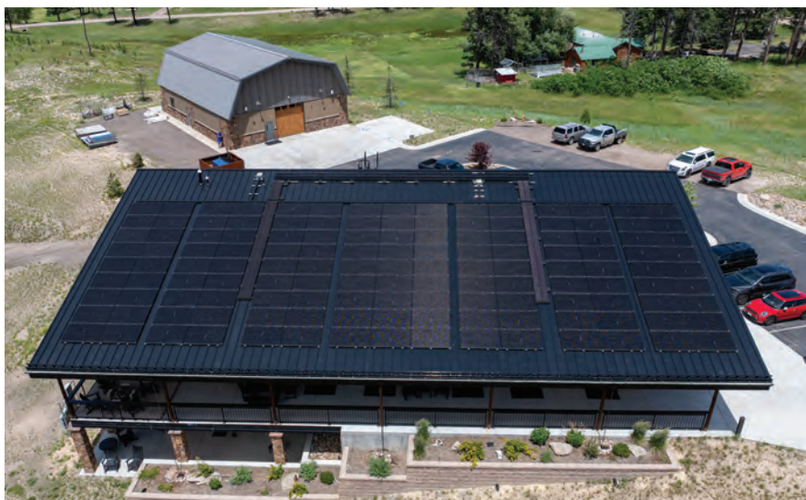
The metal roof of the S-5! corporate office is designed to allow for a 15% gap at the eave between the solar array and the snow retention system.
