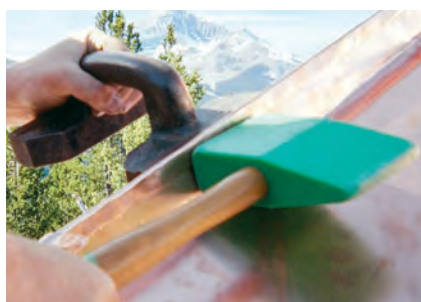
Mike Winters, owner of Mike's Metal Works in Bozeman, Montana, uses hand seamers (top) and a mallet to seam copper standing seam panels on this Montana residential jobsite. MIKE'S METAL WORKS PHOTOS
