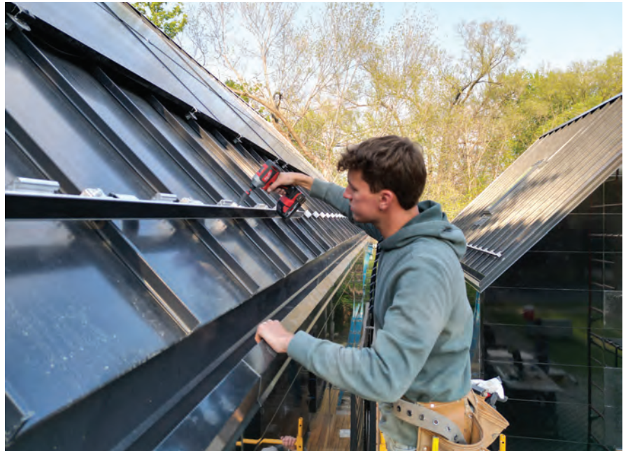
University of Kansas School of Architecture & Design student installs S-5! ColorGard® snow retention on the student-led design-build project in Lawrence, Kansas. PHOTOS COURTESY OF S-5!
