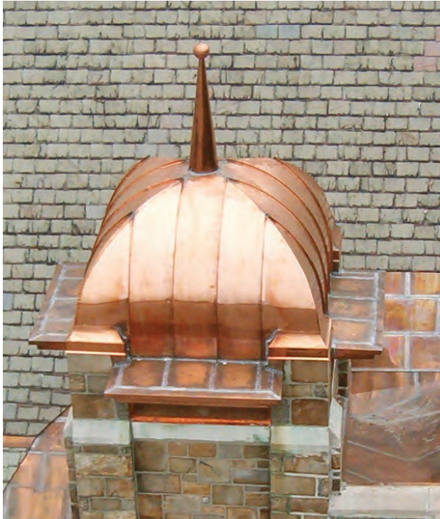
Crocker Architectural of Oxford, Massachusetts, uses hand seamers because owner David Crocker believes they do a better job, provide a tighter seal. Hand seaming also works better with specialty projects, like curved panels. CROCKER ARCHITECTURAL PHOTO
