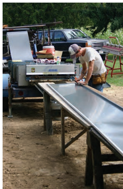
Jason Golke marks the panel where it has to be cut and folded before it is installed.
