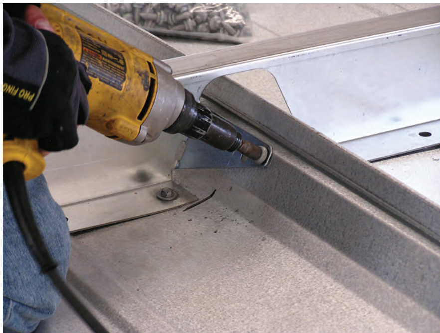
Anti-rotation arm being attached. PHOTO COURTESY OF ROOF HUGGER
