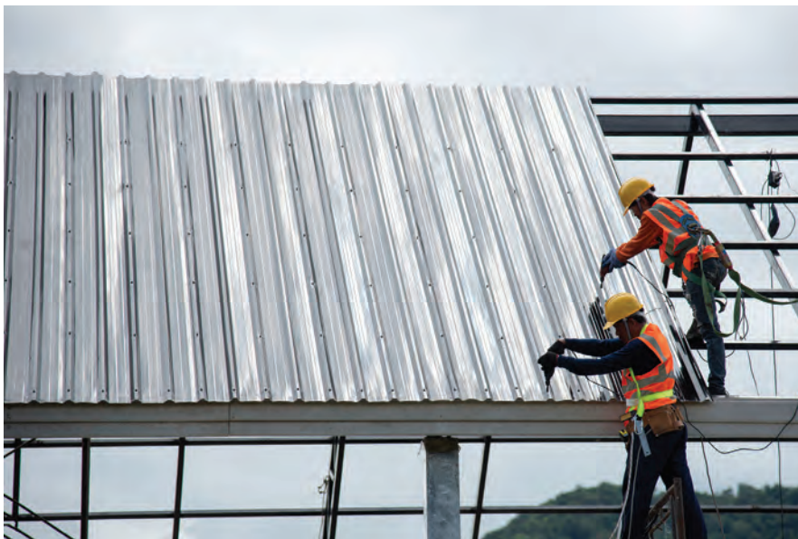
While not always true, steel purlins tend to have a firmer grip than other materials, providing a secure anchor point that allows for wider fastener spacing. PHOTO COURTESY OF TRIANGLE FASTENER CORP.
