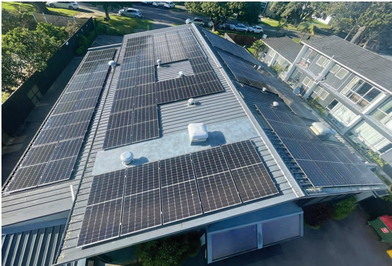
The 20-year-old roof of the McIndoe Clinic, a purpose-built consultation and day surgery facility for oral and maxillofacial surgery in the Bay of Plenty region in New Zealand, was retrofitted with a trapezoidal metal roof and a 29.5-kilowatt rooftop solar array utilizing the S-5! PVKIT rail-less solar mount.
