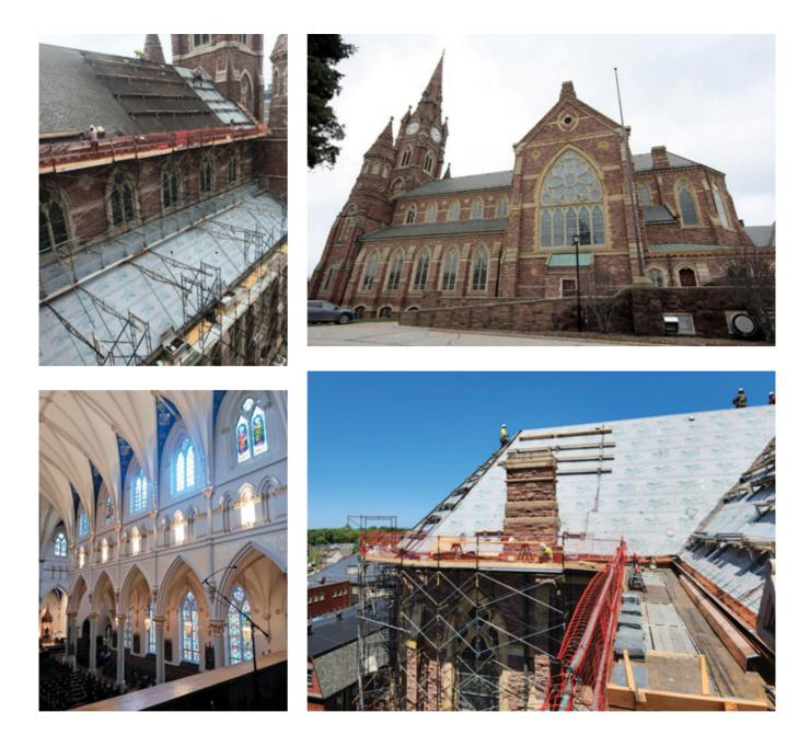
sure there are no cracks. The slate will ping in just the right way to confirm, soundness. In addition, slate was pulled from three separate pallets onto one, to maintain even color dispersion across the roof plane, to eliminate blotches of lighter and darker slates.
