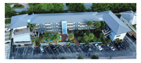
The Ocean Reef Hotel re-roofing project was a seamless transformation, showcasing the durability and sleek aesthetics of Englert's S1300 fully striated Slate Gray aluminum panels. Spanning 91 squares on a 4/12 pitch, the new metal roof replaced an aging tile system, enhancing the hotel's resilience against South Florida's coastal elements.
