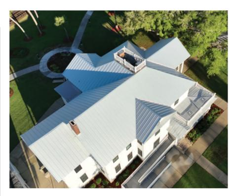
historic house re-roofed with a beautiful Galvalume Standing Seam roof by Eustis Roofing. The Clifford House, built in 1910, gets its first new roof since the original asbestos roof was installed in 1910. Once known as the Orange Capital of the World, this 18-room mansion is now used as the Eustis Historical Museum.
