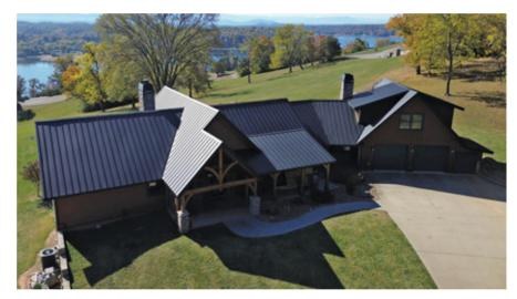
The K&L Roofing project in White Pine, Tennessee, is a stunning example of precision craftsmanship and premium materials. Spanning 5,400 square feet, this residential installation features True Metal Supply's Textured Black 26-gauge DuraLock 100 Standing Seam roofing. The striated panel design enhances long-term performance by minimizing oil canning and increasing structural integrity. Finished
