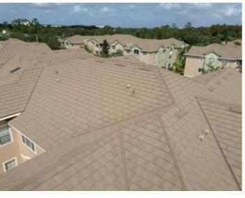
hen Orlando's Summergate Condominiums faced the need to replace their aging roof, structural limitations from a dated truss system and thin plywood made a traditional concrete tile reroof impossible. Stratus Roofing installed Unified Steel<sup>TM</sup> Stone Coated Roofing in combination with Westlake Royal<sup>TM</sup> Roofing Components' Elevated Batten System® over MetalSeal HT Underlayment, providing the perfect lightweight solution while maintaining aesthetic appeal.
