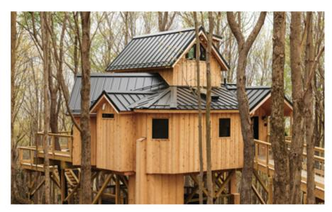
his project created some unique challenges because the terrain and trees made it difficult to get equipment in. The crew at Built Tight Builders, LLC did an amazing job using ladders and a small lift to install the roof panels. Also, the angle of the side wings created some challenging areas to flash. ShieldPro Metals was able to design custom trims to create a beautiful, watertight finished product.
