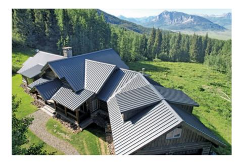
his residence is located at 10,000 ft. of elevation just outside of Crested Butte, Colorado. One aspect of the job that was especially important to the customer was reducing the likelihood of metal oil canning. To ensure a neat roof appearance and sliver the possibility of oil-canning, the contractor advocated for using a narrower
