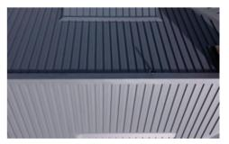
12" panel with a single added striation for rigidity. This was manufactured in 1.5" mechanical lock standing seam style. The result was a sleek and sturdy roof appearance with a success in minimal to no oil canning.
