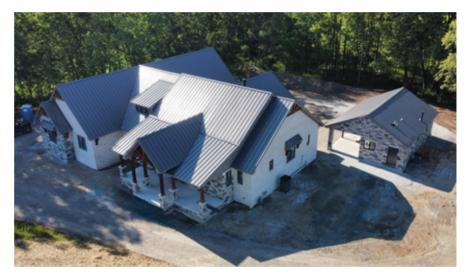
his newly constructed home in Brownsburg, Indiana, was completed with a lifetime standing seam metal roof. MP150 standing seam metal panels with hemmed and riveted trim were made on site with a New Tech Machinery roll former rented from Indiana Metal.
