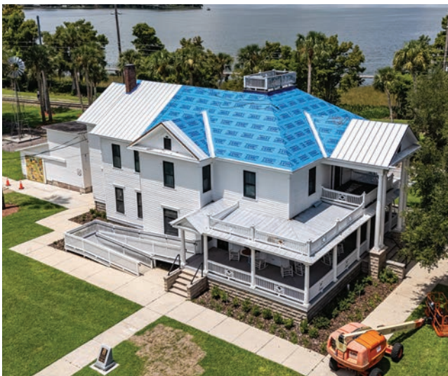
During re-roofing process.
