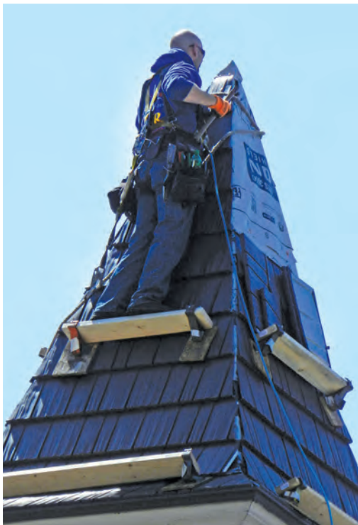
Metal's relatively low weight makes it a great choice for steep-slope installations.
