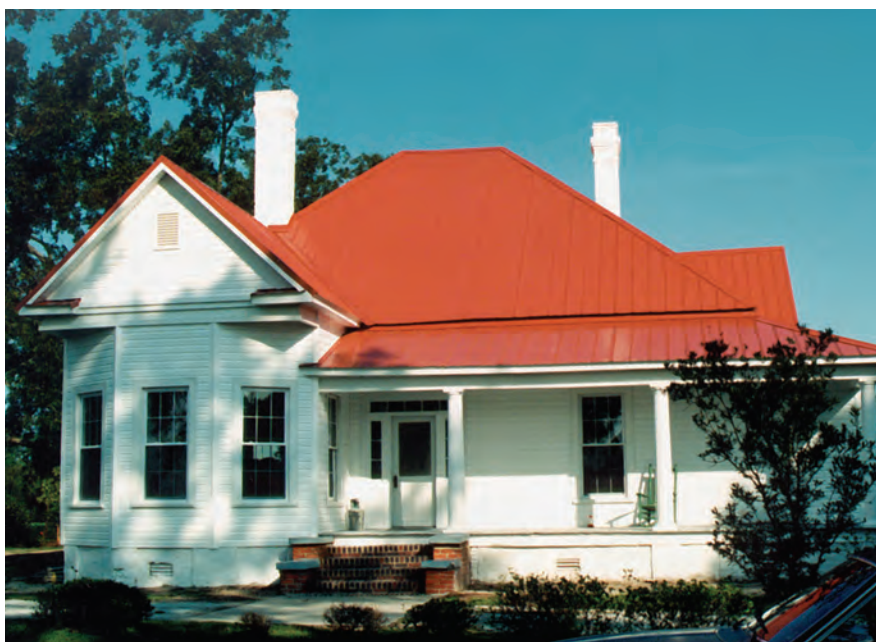
Some homeowners have discovered that 5-v crimp roofing is an economical alternative to mechanically seamed standing seam roofing. They get many of the same benefits and aesthetics, only with an exposed fastener. FABRAL PHOTO
