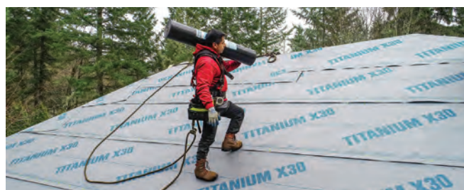
Titanium X30 underlayment. PHOTO COURTESY OF OWENS CORNING/TITANIUM
