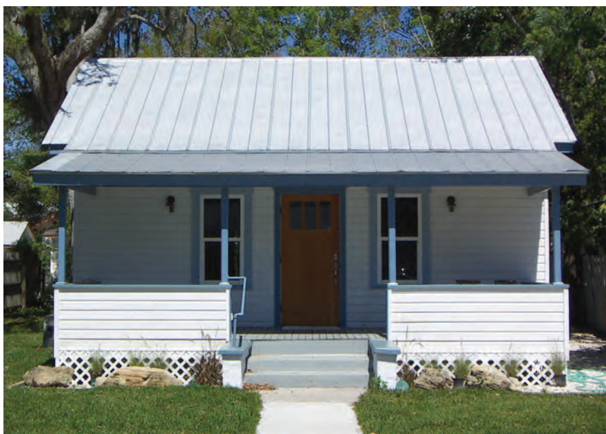
This residence in New Smyrna Beach, Fla., was recently re-roofed in 5-v Galvalume. It is a 750-square foot wood-frame Cracker shotgun, with two bedrooms and one bath, built in 1918. The roof, installed as part of a complete renovation, is sloped at 4:12 with 5-v installed over 1x4 sleepers over 2-inch rigid insulation over the existing 1x4 heartpine decking. ARCHDESIGN PHOTOS
