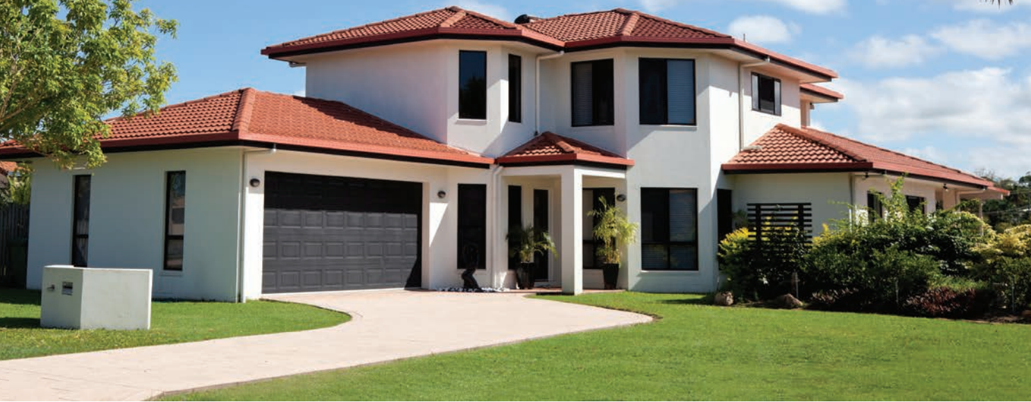
The characteristics of high-quality metal roofs make them suitable for today's long-lasting solar systems. PHOTO COURTESY OF PPG.
