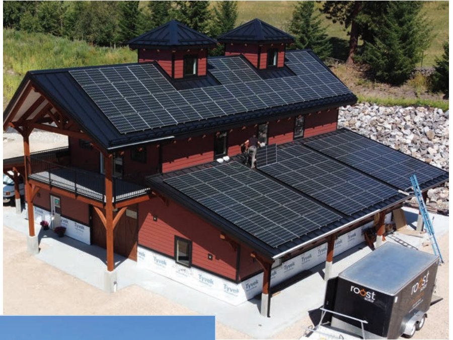
With an 8:12 roof pitch, the design and installation of both the solar modules and snow guard systems were effectively coordinated for this equestrian estate in Vernon, British Columbia, Canada. PHOTOS COURTESY OF S-5!
