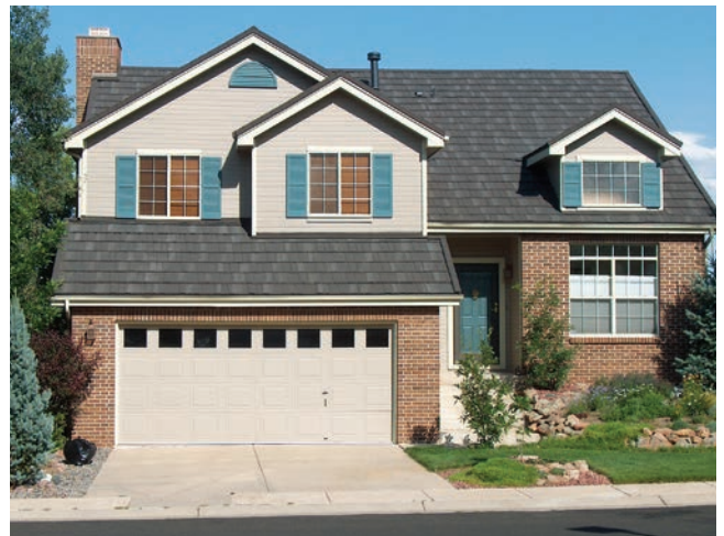
DURA-LOC ROOFING PHOTO
