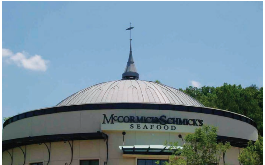
A very complex roof combining double lock standing seam and the batten cap method was used on McCormick and Schmick Seafood Restaurant in Birmingham, Ala. It was specified by Boora Architects and installed by Ornametals. Zinc roofing by Umicore was used not only due to its appealing aspect, but also because it is very flexible metal.
