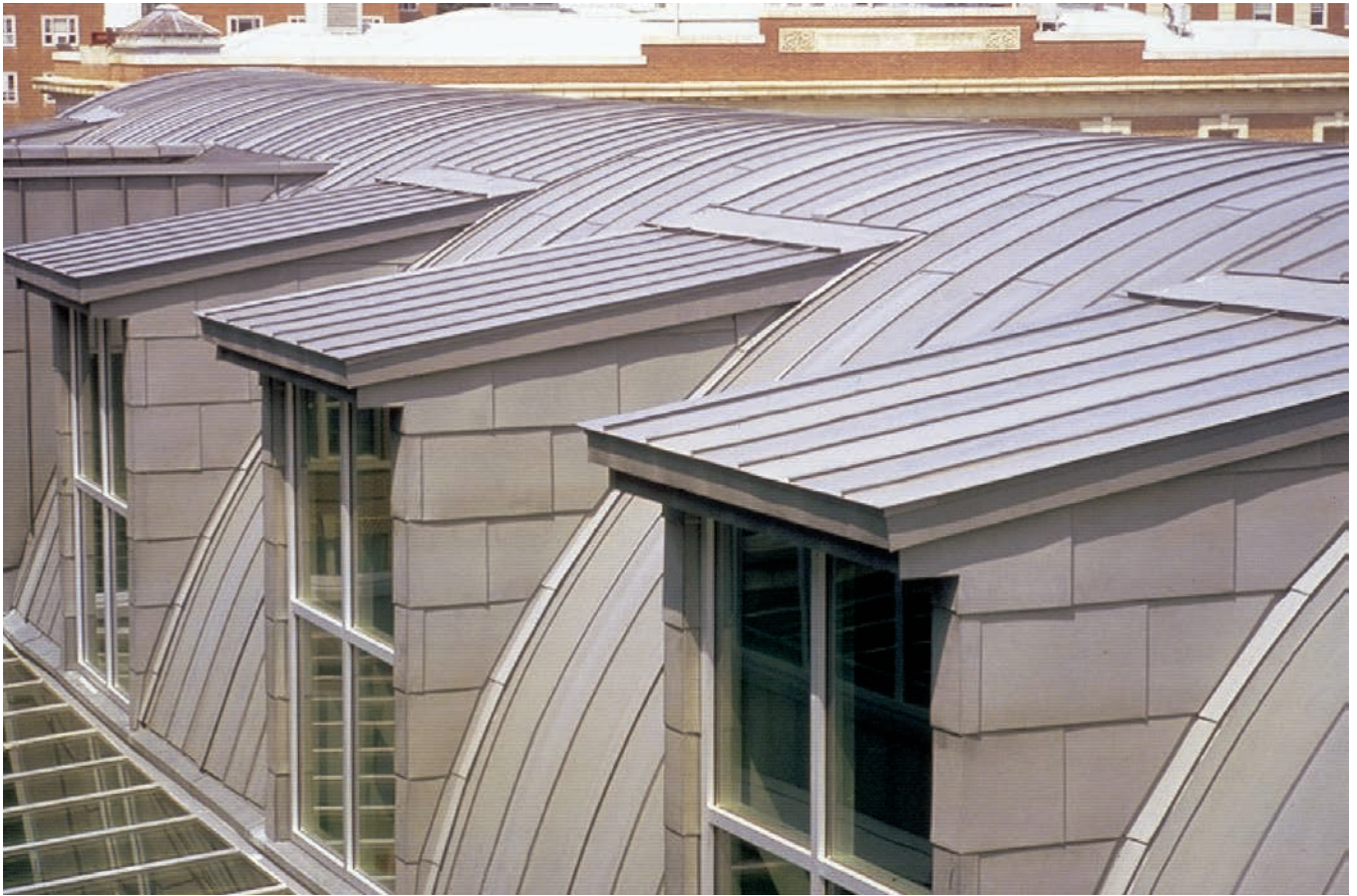
Because zinc is an even more malleable than steel or aluminum, it can be curved and formed easily while still providing a watertight roofing system. VM ZINC PHOTO
