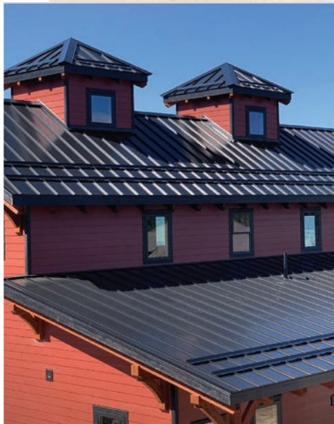
With an 8:12 roof pitch, the design and installation of both the solar modules and snow guard systems were effectively coordinated for this equestrian estate in Vernon, British Columbia, Canada. PHOTOS COURTESY OF S-5!
