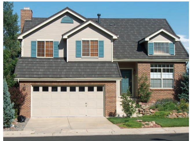
DURA-LOC ROOFING PHOTO
