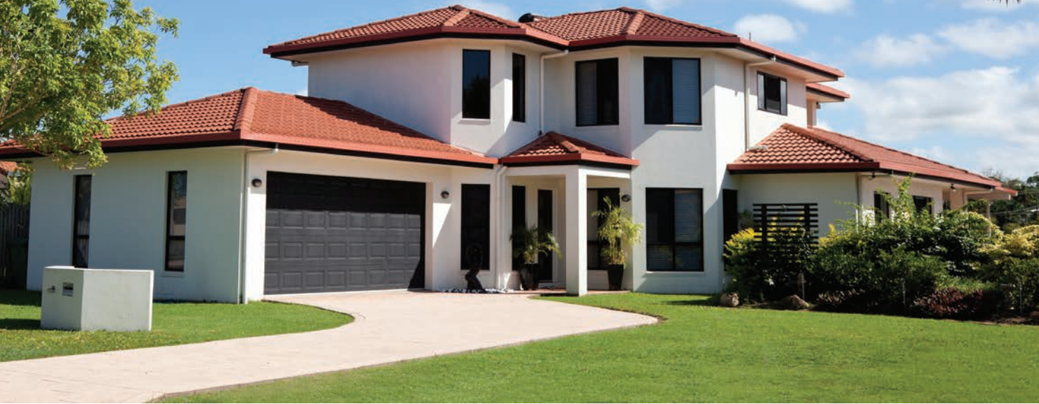
The characteristics of high-quality metal roofs make them suitable for today's long-lasting solar systems. PHOTO COURTESY OF PPG.
