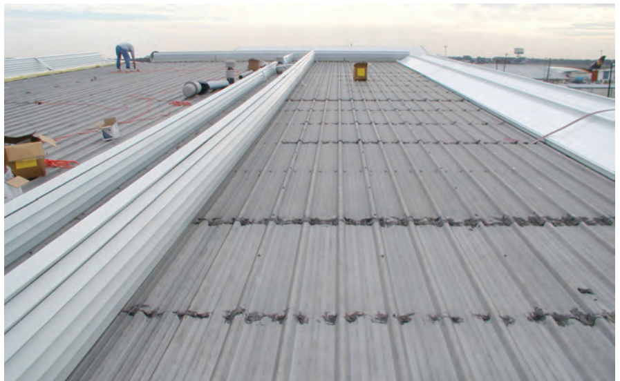
Miller Roofing of Lafayette, La., installed 16,700 square feet of roofing over 9,200 linear feet of The Roof Hugger on the Aviation Maintenance Technology Building at Louisiana Technical College. The panels, manufactured by Architectural Building Components of Houston, were 22 inches wide and 101 feet long. ARCHITECTURAL BUILDING COMPONENTS PHOTOS
