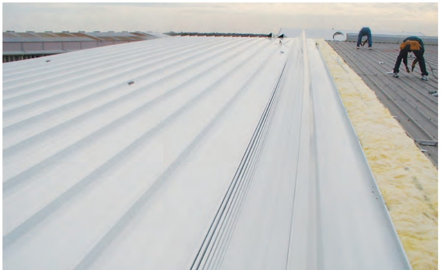
Miller Roofing of Lafayette, La., installed 16,700 square feet of roofing over 9,200 linear feet of The Roof Hugger on the Aviation Maintenance Technology Building at Louisiana Technical College. The panels, manufactured by Architectural Building Components of Houston, were 22 inches wide and 101 feet long. ARCHITECTURAL BUILDING COMPONENTS PHOTOS
