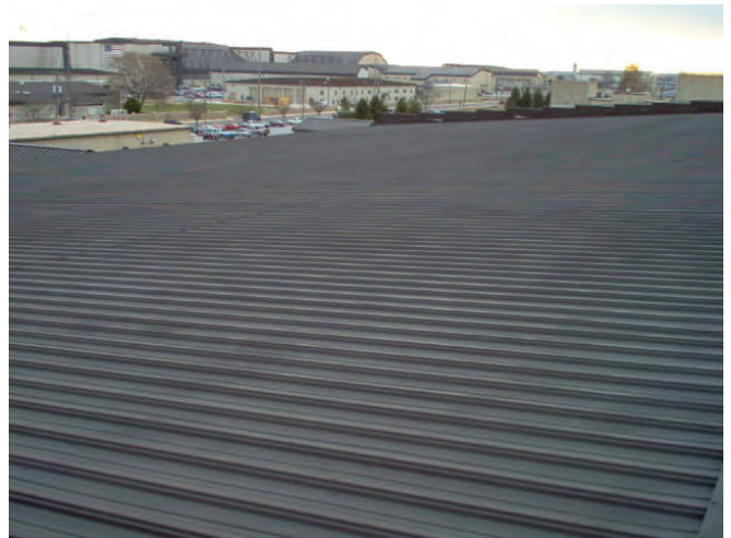
Interstate Panel of Hamilton, N.J., installed 9.75 miles (51,500 linear feet) of the Roof Hugger for a military project in Dover, Del. Roof Hugger spacing in the field of the roof is every 5 feet on center. Spacing on the perimeters is every 2-1/2 feet on center. A 2-inch isocyanurate board insulation was installed between the Roof Huggers. The project called for more than 28.7 miles (210,000 square feet) of 22-gauge Ultra Seam US200 mechanically seamed panels. BALLARD BUILDERS PHOTOS
