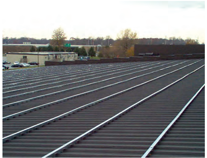
Interstate Panel of Hamilton, N.J., installed 9.75 miles (51,500 linear feet) of the Roof Hugger for a military project in Dover, Del. Roof Hugger spacing in the field of the roof is every 5 feet on center. Spacing on the perimeters is every 2-1/2 feet on center. A 2-inch isocyanurate board insulation was installed between the Roof Huggers. The project called for more than 28.7 miles (210,000 square feet) of 22-gauge Ultra Seam US200 mechanically seamed panels. BALLARD BUILDERS PHOTOS
