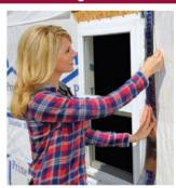
Extend your building season with WindowWrap PowerBond adhesive system, which aggressively adheres in cold weather down to 25° F, while remaining stable at elevated temperatures. It features a flex option for sill pan flashing and curved openings, self-seals around common fasteners, is more economical than butyl-based products, and is made in the USA.
