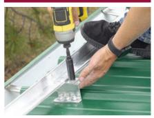
VersaBracket is a bottom-fixed, metal roof bracket designed for mounting ColorGard, solar PV, and other utility mountings to exposed fastened profiles. VersaBracket features a 1" mounting slot on the top flange for adjustability and fastens through the roof, into the deck or structure. Factory-applied butyl sealant ensures speedy installation and lifetime performance.
