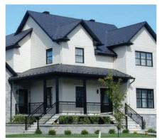
Wakefield Bridge long-lasting steel roofing panels are manufactured in compliance with the High Velocity Hurricane Zone provisions of the Florida Building Code and are designed to resist high winds (TAS100, Miami-Dade, 140mph) and burning embers (fire-rated class A. ASTM E108).
