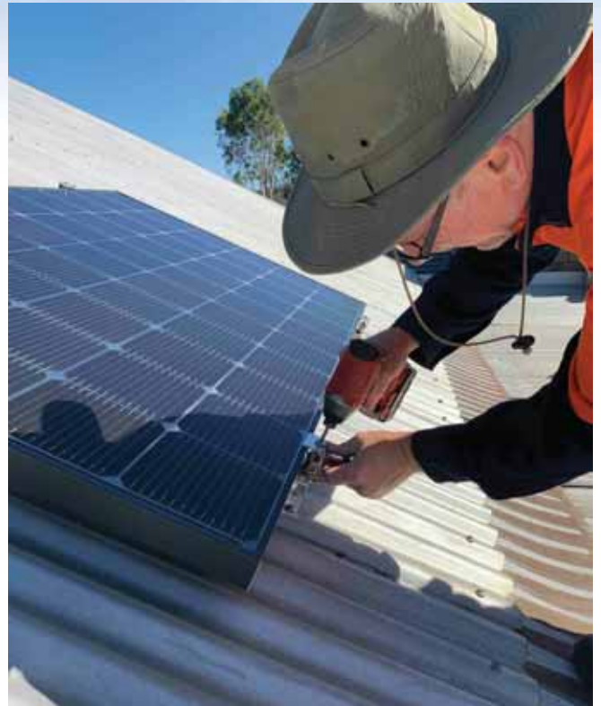
Installing an S-5! PVKIT™. PHOTO COURTESY OF S-5!
