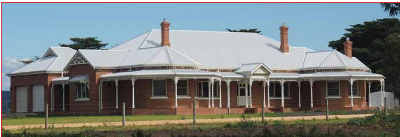
Corrugated residential roofing installed 20 years ago. PHOTO COURTESY OF APPLICAD, AUSTRALIA
