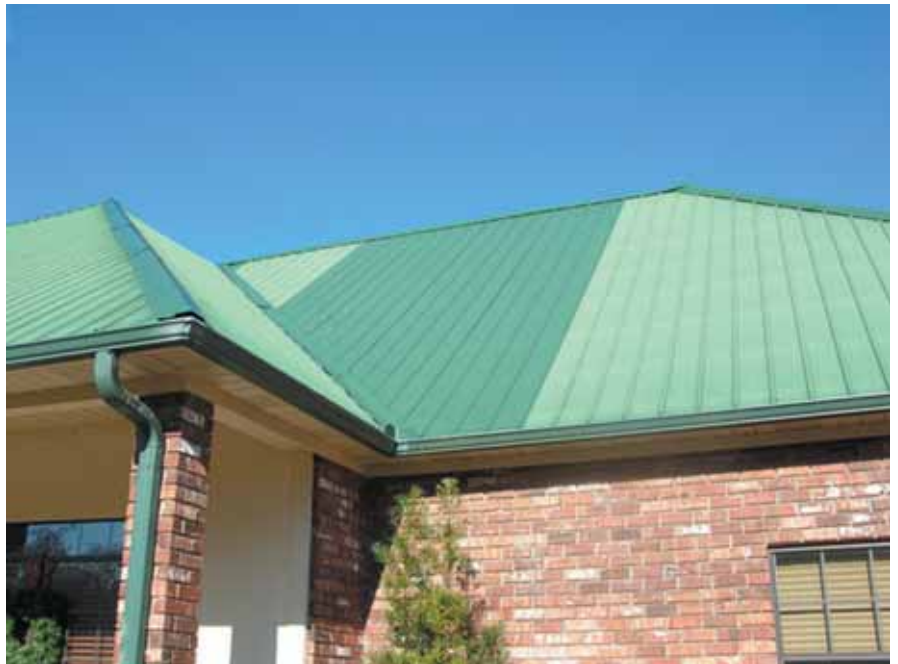
Some manufacturers may state a long warranty coverage yet allow great degrees of color and chalk. PHOTO COURTESY MCELROY METAL.
