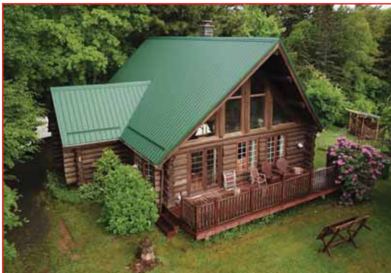
Corrugated residential roofing. PHOTO COURTESY OF WALL ROOFING, NOVA SCOTIA
