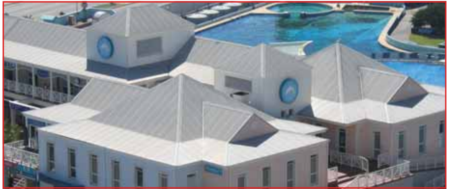
Commercial roof in a corrugated, painted profile. PHOTO COURTESY OF APPLICAD, AUSTRALIA
