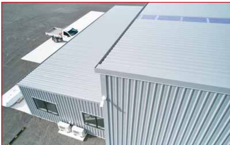
Commercial roof and wall cladding in trapezoidal profile. PHOTO COURTESY OF THE RIVERLEA GROUP, NEW ZEALAND
