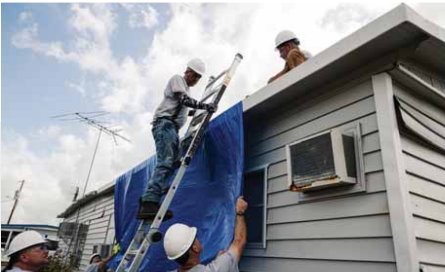
Hurricane response in Florida.
