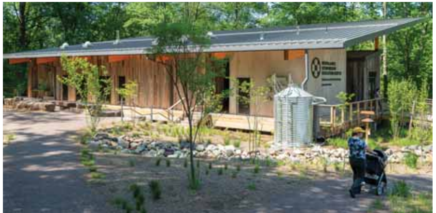
Metal Sales Manufacturing Magna Lock 180 / Flush Seam tops the Woodlands Stewardship Education Center in Chantilly, Virginia. PHOTO COURTESY OF QUINN EVANS ARCHITECTS.
