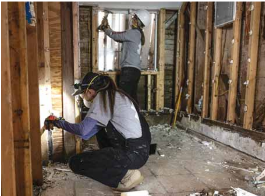
Flooding response in San Diego. PHOTOS COURTESY OF TEAM RUBICON.
