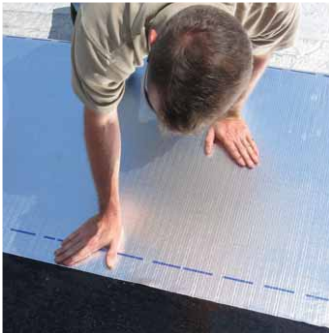
Peel & Seal® features an embossed aluminum surface that can be exposed to the elements indefinitely without the use of specialty coatings.
