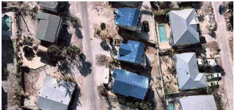
Cape Coral image after damage-causing weather event, showing temporary roof repairs.
