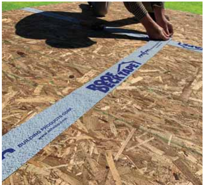
Roof Deck Tape® adds another layer of waterproofing protection to plywood and OSB roof panels.
