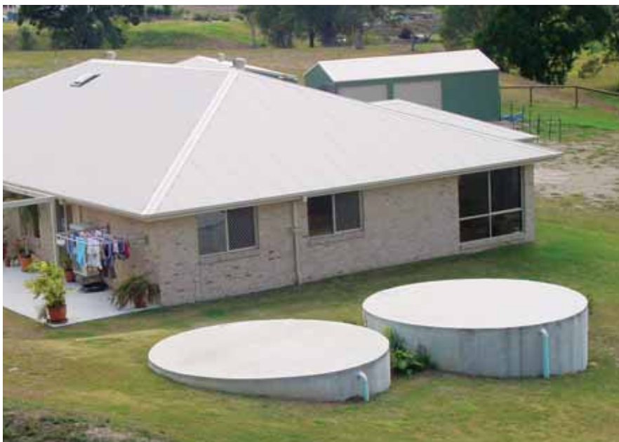
Rain water harvesting is an ancient practice making a resurgence in many areas, and modern systems work best with metal roofing systems. JIM RYAN PHOTOS
