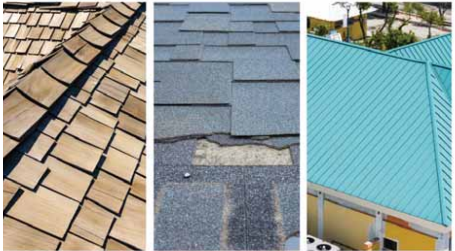
Metal roofs reflect heat, last longer, and require less maintenance.
