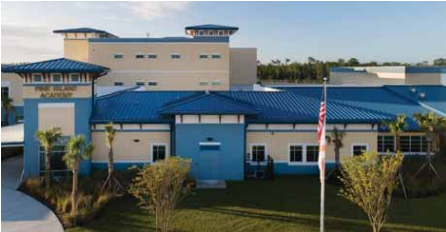
St. Augustine, Florida's Pine Island Academy is roofed primarily in low-rise membrane. However, sloped metal accents of PAC-CLAD metal roof panels help break up the façade and add interest to the roofline. PHOTO BY HORTONPHOTOINC.COM
