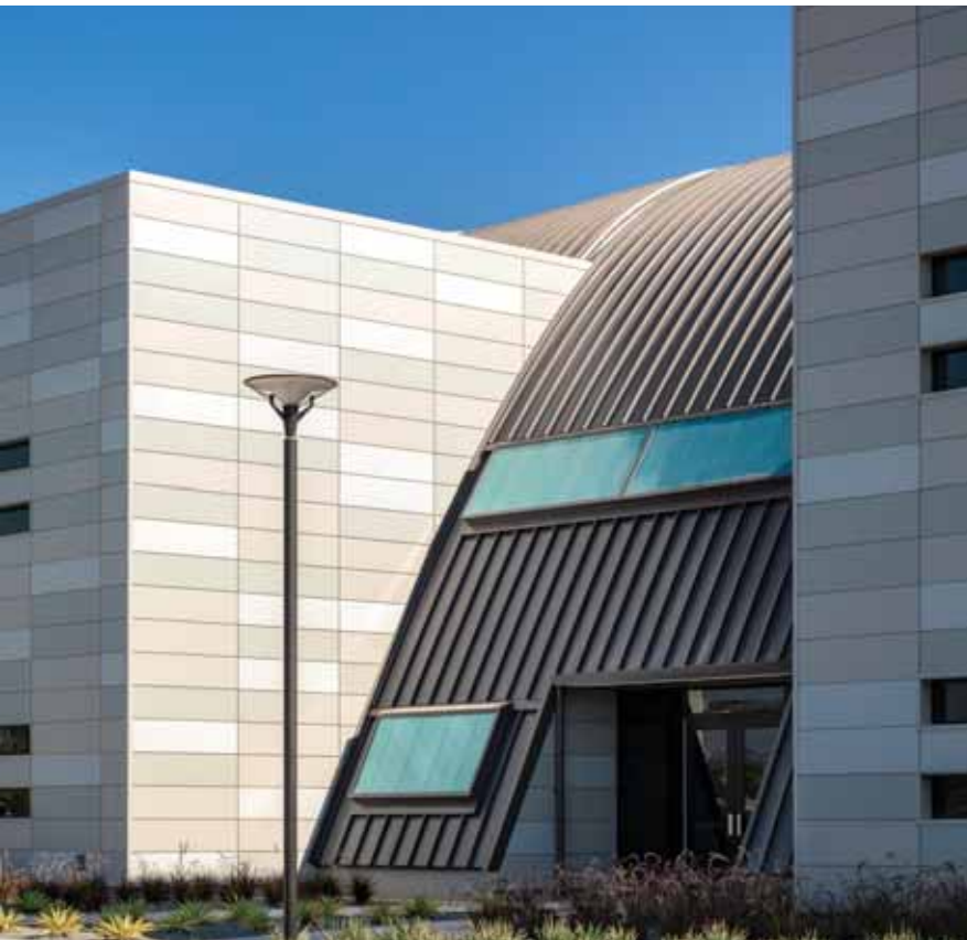
Tustin Legacy Magnet School in Tustin, California, is a TIDE (technology, innovation, design, entrepreneurship) focused 6-12th grade campus. The exterior is finished in Dri-Design Painted Aluminum Panels. PHOTO COURTESY @RMA PHOTOGRAPHY INC.
