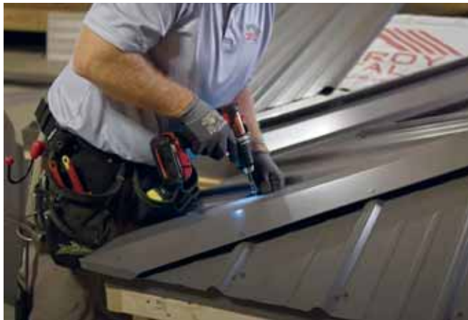
Screw guns with an adjustable clutch are the preferred installation tool for self-drilling fasteners. IMAGES COURTESY OF MCELROY METAL.
