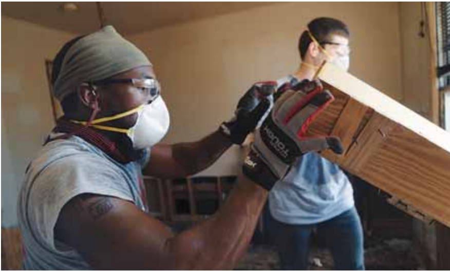
Rebuilding in Selma, Alabama. PHOTOS COURTESY OF TEAM RUBICON.
