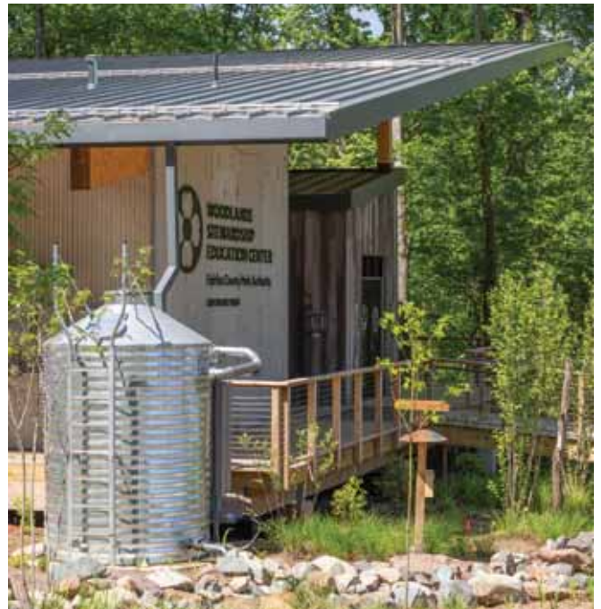
Rain is collected off the metal roof of the Woodlands Stewardship Education Center in Chantilly, Virginia.. PHOTO COURTESY OF QUINN EVANS ARCHITECTS.
