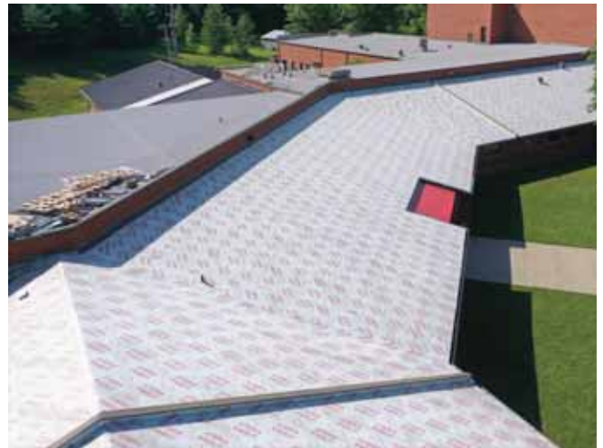
MFM products are self-sealing around construction fasteners to maintain a complete waterproof barrier.
