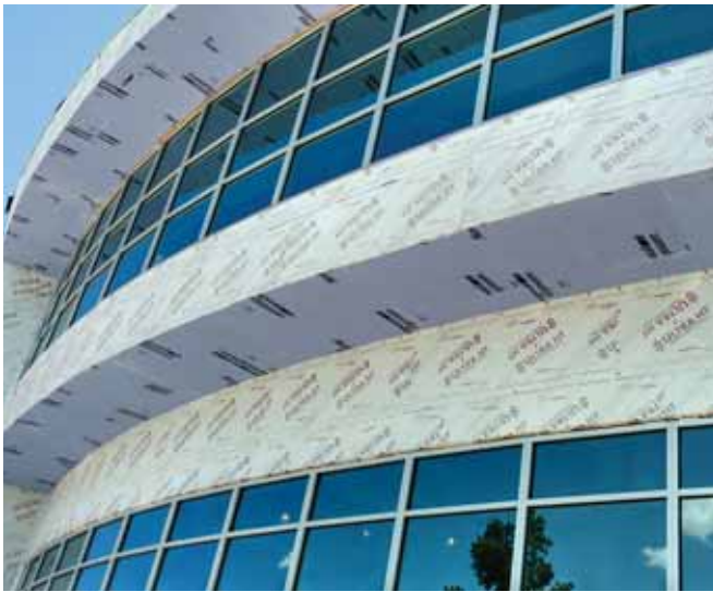
Ultra HT Wind & Water Seal® is a high-temperature rated underlayment that can be used beneath metal side panel systems as a vertical flashing membrane. PHOTOS COURTESY OF MFM
