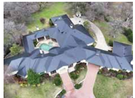
Roof after replacement
