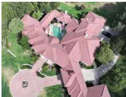
Roof before replacement
