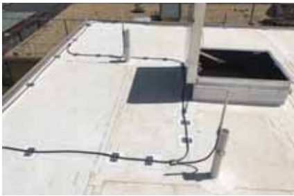
Lightning protection conductors must be securely fastened and bends must be gradual to ensure that the lightning current can travel easily within the lightning protection system.
