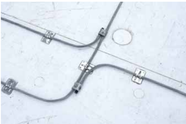
Lightning protection standards contain specific requirements for conductor coursings, fastener placement and interconnection methods for joining conductors and building systems. Photos courtesy of East Coast Lightning Equipment, Inc.
