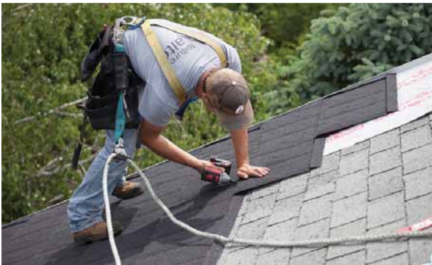
Installation of Metstar M.I.T. stone-coated steel shingles. COURTESY OF METSTAR M.I.T.
