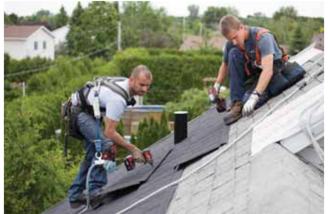
Installation of Metstar M.I.T. stone-coated steel panels. COURTESY OF METSTAR M.I.T.
