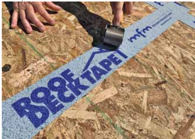
MFM Roof Deck Tape™ is designed to effectively seal the seams on plywood and OSB roofing panels. Cover with any of MFM's underlayment products for complete waterproofing protection! Watch the video on our website.
