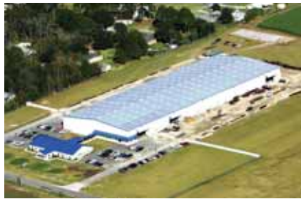
Ideal Steel headquarters, Broussard, Louisiana.
