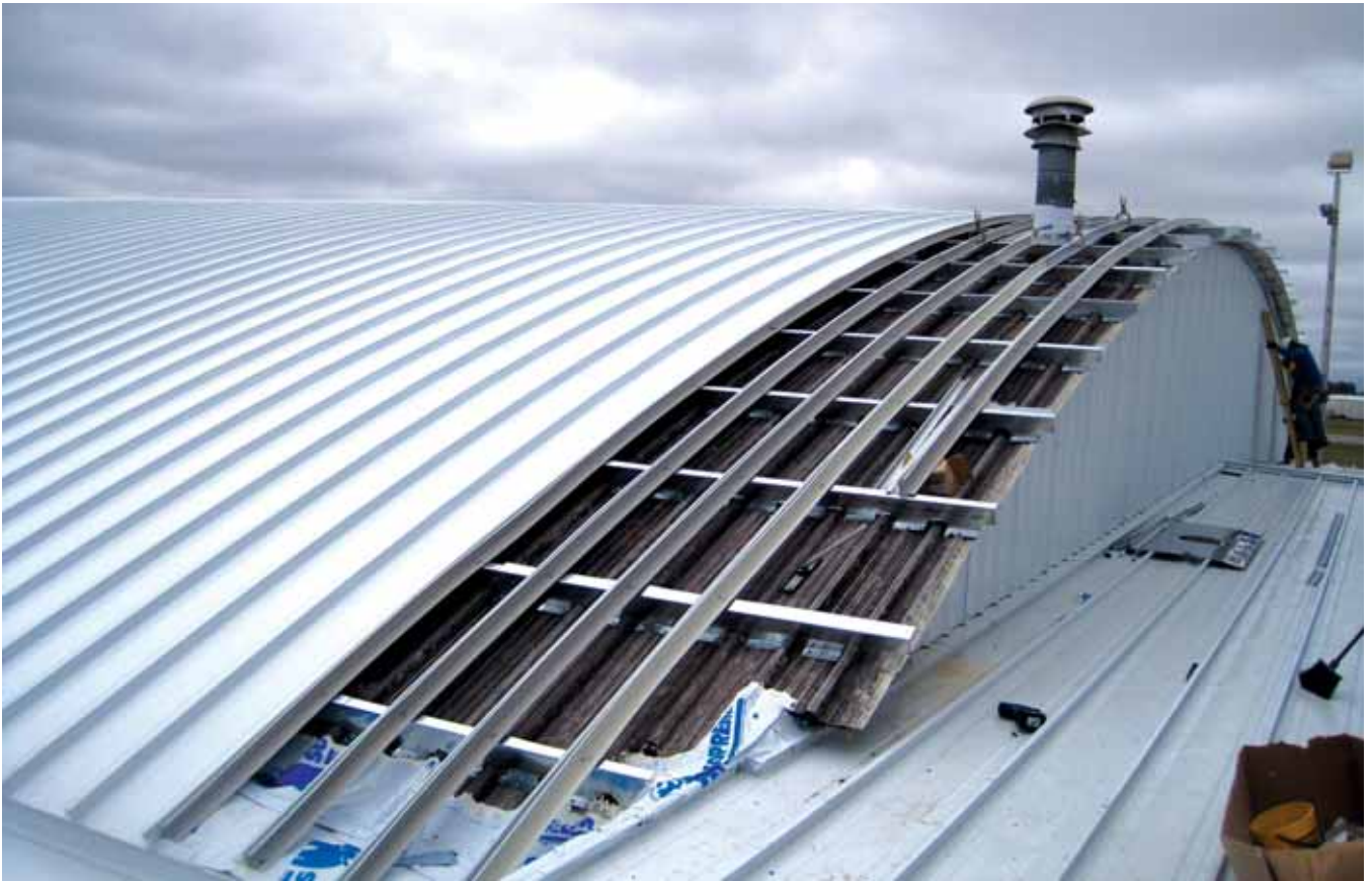
Metal-over-metal can be installed over a curved roof. PHOTO COURTESY OF ROOF HUGGER
