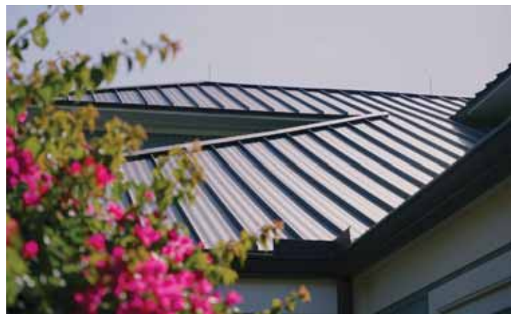
The DMC 175S profile used features a 1¼" seam height and in this instance, a 16" panel width. The metal panels were finished in Inkwell, a low-gloss dark charcoal-gray color, to reduce glare for the golfers. PHOTOS COURTESY OF DREXEL METALS.
