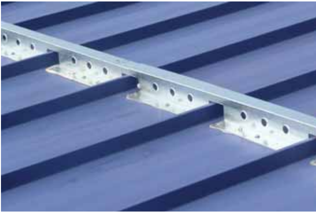
Vented Roof Hugger installed over standing seam panels.
