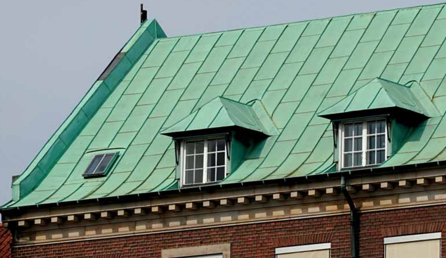
Copper roof with patina.
