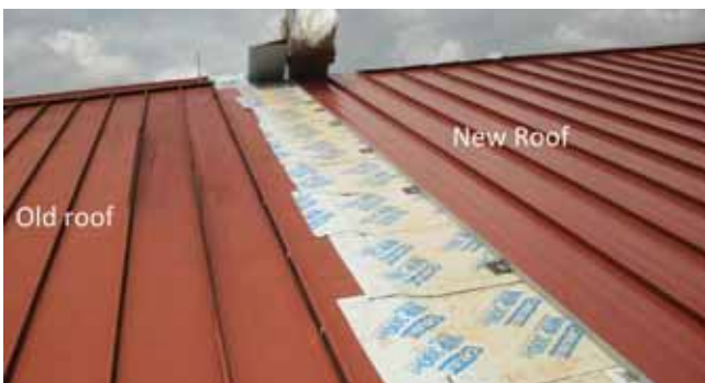
Colors may come close, but it is difficult to get exact matches without ordering custom. PHOTO COURTESY OF PAC-CLAD | PETERSEN
