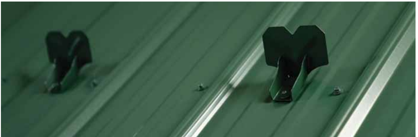
Snow guards are attached using the roof panel fasteners on through-fastened panels. PHOTO COURTESY LEVI'S BUILDING COMPONENTS
