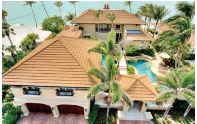
This coastal home features Unified Steel Stone Coated Pine Crest Shake. PHOTO COURTESY OF UNIFIED STEEL/MRA
