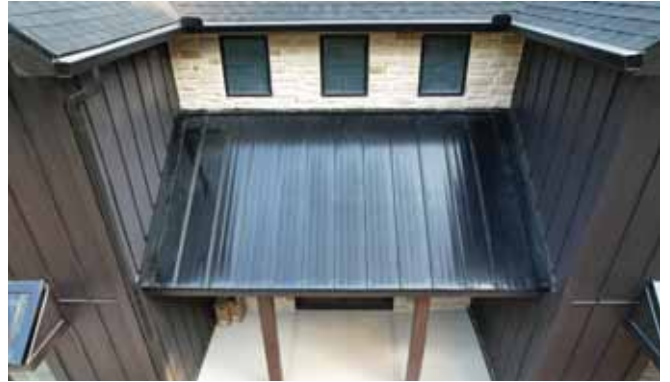
If roof areas requiring replacement can be easily sectioned, standing seam metal roofing provides a beautiful accent. It complements many roofing styles and textures, making it an excellent option for renovations. DuraLock™ Standing Seam (shown) manufactured by True Metal Supply. PHOTOS COURTESY OF FLOW ROOFING.
