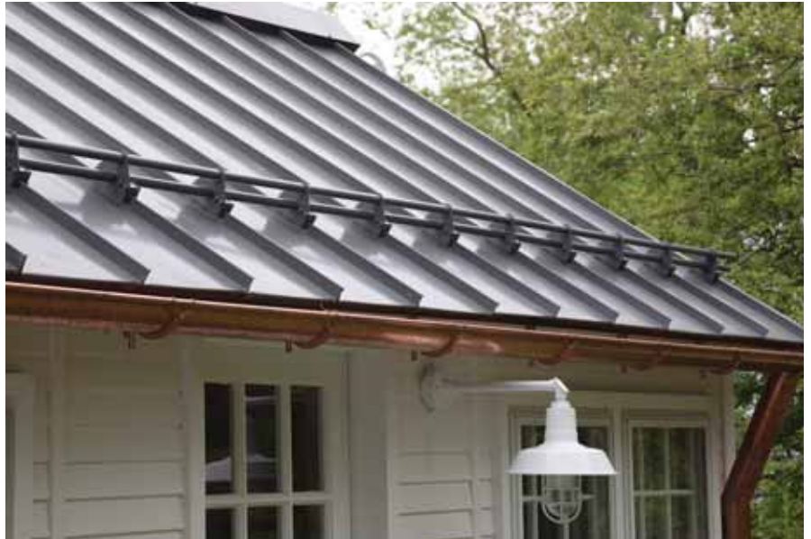
A continuous snow guard system keeps heavy, wet snow from sliding down onto whatever — or whomever — is beneath the eaves. PHOTO COURTESY OF S-5!
