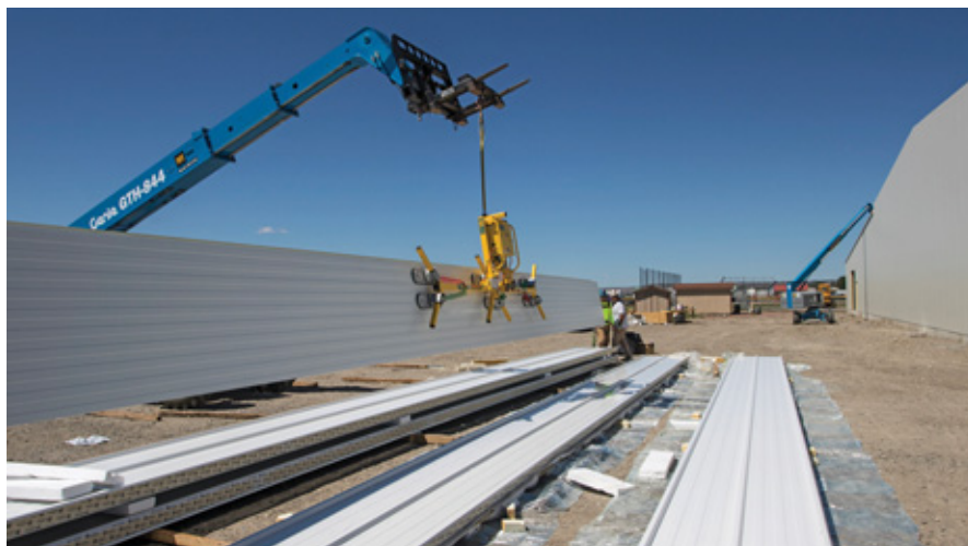
Vacuum suction cup lifting, popular in Europe, is now commercially available in the U.S. Courtesy of Wood's Powr-Grip
