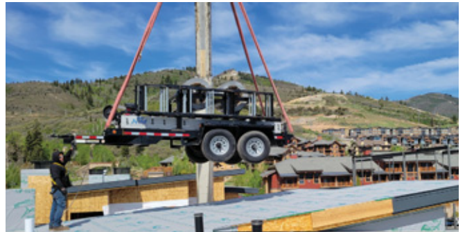
If needing to lift your machine to roof height you'll want an open flatbed like this Maxey Trailer owned by Homie Mulcahy of SaltedMetals in Utah. PHOTO COURTESY OF SALTEDMETALS ARCHITECTURAL METALS DESIGN AND CONSULTING
