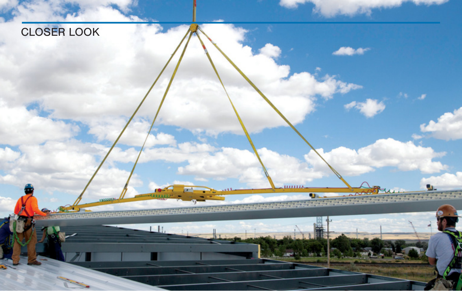
To ensure optimized performance and aesthetics, insulated metal panel wall and roofing systems must be carefully stored, transported, and lifted. Courtesy of Wood's Powr-Grip
