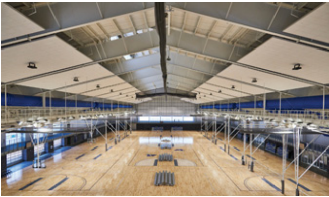
According to a recent MCA study, coated standing seam roofing systems have a service life of 60+ years, which is far longer than the average PV array service life of 32 1/2 years. CFR roof panels installed in the Finley Center, part of the Hoover Met Complex, Hoover, Alabama. PHOTO COURTESY OF NUCOR/METL SPAN.
