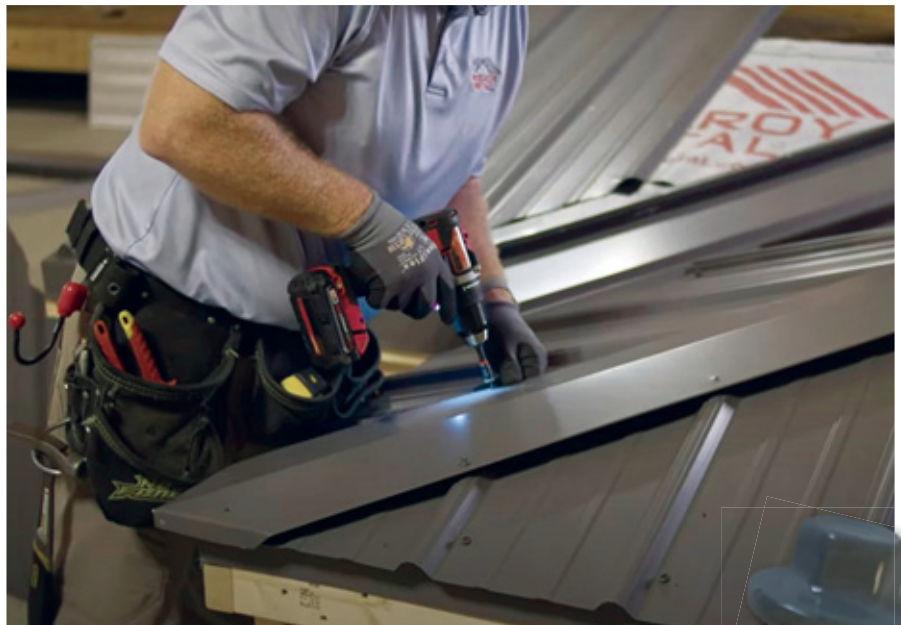
Practicing installation of exposed fastener metal panels and trims. PHOTO COURTESY OF MCELROY METAL
