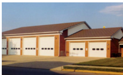
A Rustic Shingle aluminum shake was selected for this fire department in Piqua, Ohio. It features reflective coatings, called Hi-R Finish by Classic Products. CLASSIC PRODUCTS PHOTO
