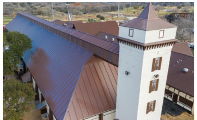
After fire damaged the Wursthof facility in New Braunfels, Texas, a new roof was needed fast. Insulated metal panels (IMPs) were specified. IMPs are faster to install than other materials for walls and roofing. PHOTO COURTESY OF NUCOR/METL SPAN.
