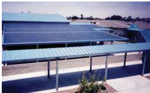
At far right, installers field-laminate the thin-film PV material onto a metal roofing panel before its installation as part of a metal roof. The material works as well on structural panels (on awnings at the Mendoza Elementary School, Imperial Beach, Calif., left) as on architectural panels (Top: on the Nature Conservancy's Conservation Learning Center near Orlando, Fla.). TOP AND TOP RIGHT, UNI-SOLAR; RIGHT: GEORGE KOTT/CHROMA
