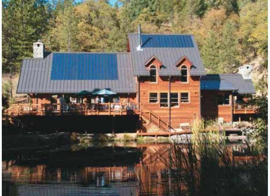
Two different applications, two different styles of photovoltaics. A residence in Northern California sports an architecturally discreet 4-kilowatt thin-film laminate solar panel, made by Uni-Solar, on its standing seam metal roof; installation by DC Power. At left, a 340 kW crystalline module PV system, made by Solarex (now BP Solar), installed on the vaulted metal roof of the main swimming facility for the 1996 Atlanta Olympics, at the time the world's largest building-based PV system. DANIEL MARINO
