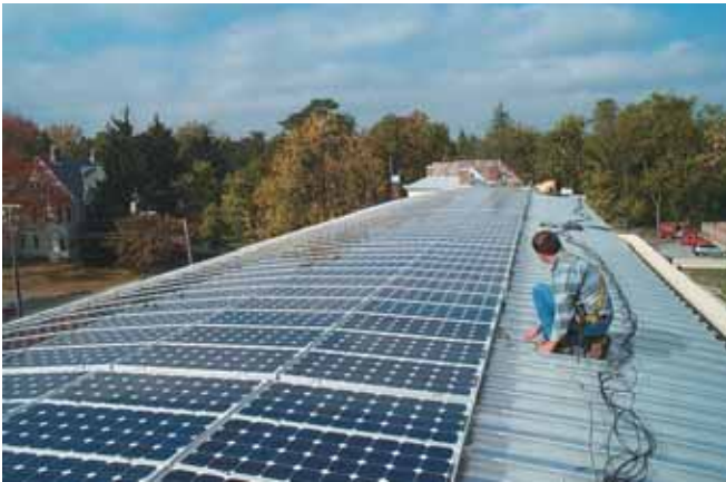
This installation at Oberlin College, on a Zip-Rib roof manufacture by Merchant & Evans, was one of the first to use a rated clip – the S5!, designed specifically for that panel profile. Below: Several styles of the S5!, and artwork detailing the standing seam PV detail. BP SOLAR, METAL ROOF INNOVATIONS PHOTOS
