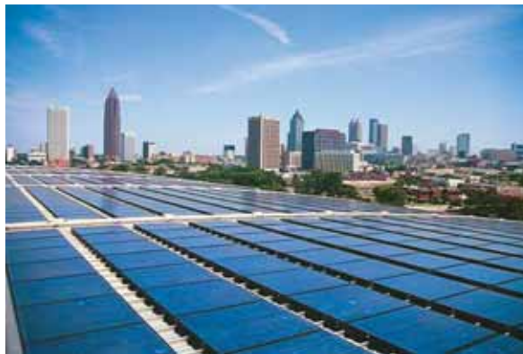
Two different applications, two different styles of photovoltaics. A residence in Northern California sports an architecturally discreet 4-kilowatt thin-film laminate solar panel, made by Uni-Solar, on its standing seam metal roof; installation by DC Power. At left, a 340 kW crystalline module PV system, made by Solarex (now BP Solar), installed on the vaulted metal roof of the main swimming facility for the 1996 Atlanta Olympics, at the time the world's largest building-based PV system. DANIEL MARINO
