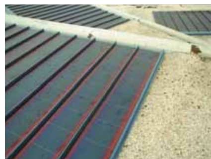
Tibor Fischl of Renewable Energy Resources used standing seam panels laminated with PV material on a flat ballasted roof in Oakland. PHOTOS © RENEWABLE ENERGY RESOURCES
