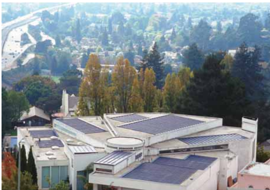
Tibor Fischl of Renewable Energy Resources used standing seam panels laminated with PV material on a flat ballasted roof in Oakland. PHOTOS © RENEWABLE ENERGY RESOURCES
