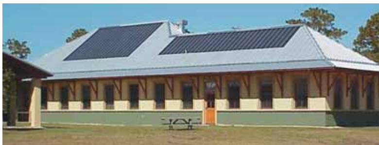
At far right, installers field-laminate the thin-film PV material onto a metal roofing panel before its installation as part of a metal roof. The material works as well on structural panels (on awnings at the Mendoza Elementary School, Imperial Beach, Calif., left) as on architectural panels (Top: on the Nature Conservancy's Conservation Learning Center near Orlando, Fla.). TOP AND TOP RIGHT, UNI-SOLAR; RIGHT: GEORGE KOTT/CHROMA
