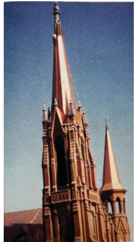
St. Augustine's in Austin, Minn., got the works: new copper shingle cladding for its steeples and a new copper standing seam roof.
