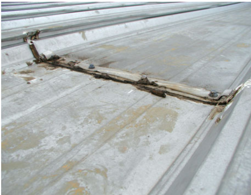
A problematic, leak prone lap on a trapezoidal standing seam.
