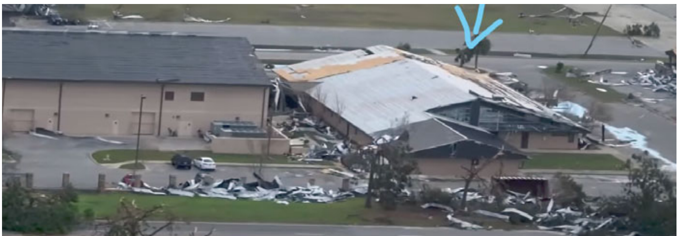
Tyndal Air Force Base, 2018: 200 mile per hour winds blew off much of the incomplete roof, but the Sharkskin underlayment remained in place.
