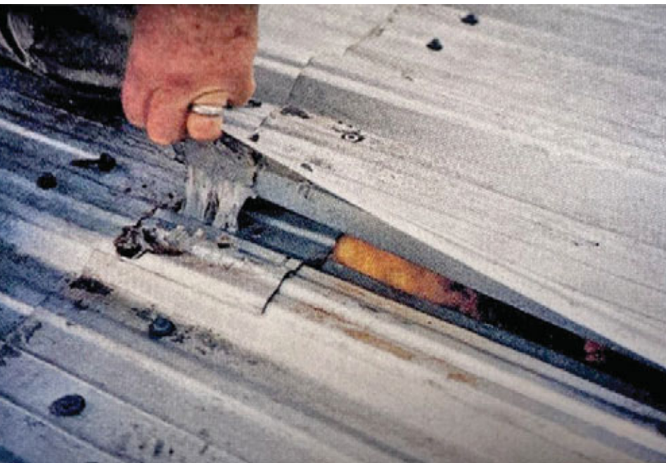
Although the end lap sealant remains effective, the absence of any side lap sealant on this roof resulted in extensive interior damage.
