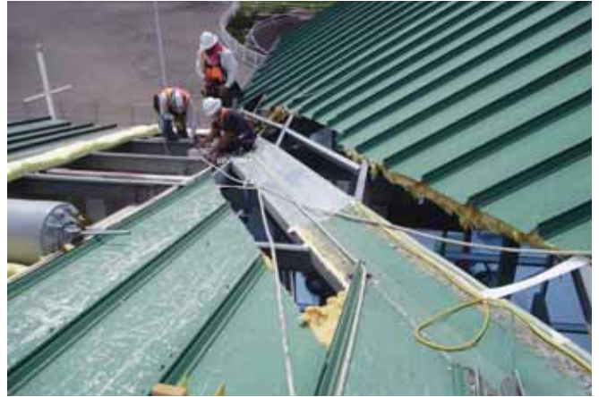
Removing and replacing the standing seam panels on a roof with an open frame. PHOTO COURTESY OF MCELROY METAL
