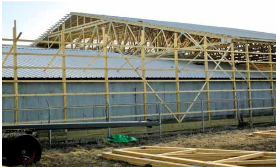
H&D Quality Builders constructs a post-frame building around and over an existing structure. PHOTO COURTESY H&D QUALITY BUILDERS
