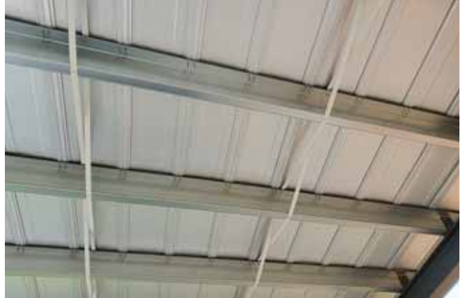
Purlin Strapping. PHOTO COURTESY OF MCELROY METAL
