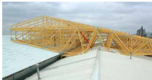
H&D Quality Builders constructs a post-frame building around and over an existing structure. PHOTO COURTESY H&D QUALITY BUILDERS
