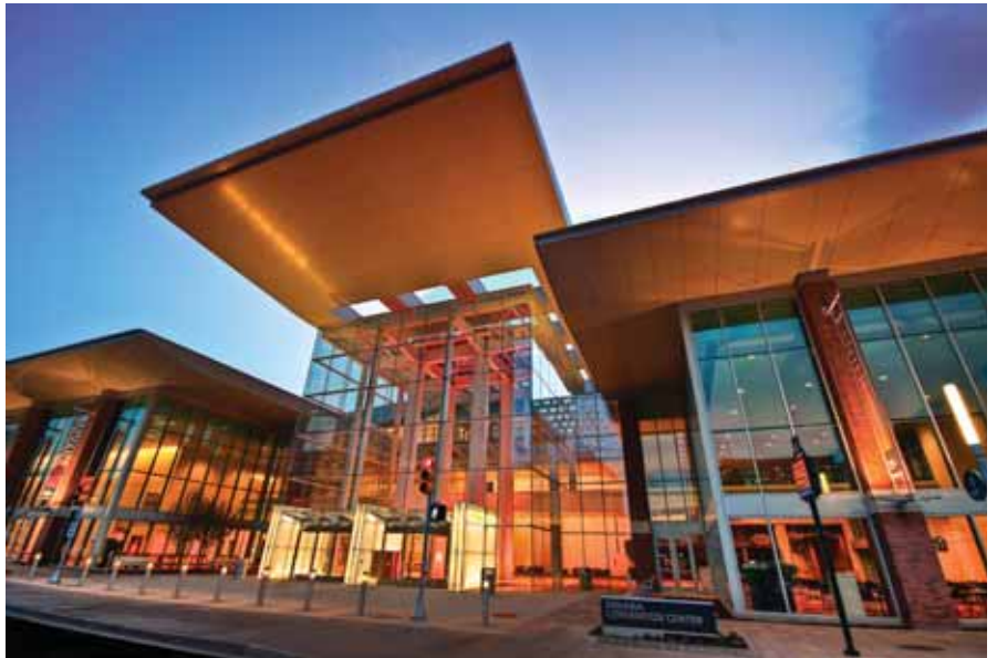
The METALCON 2022 trade show takes place Oct. 12-14 at the Indiana Convention Center in Indianapolis. Photo courtesy of the Indiana Convention Center
