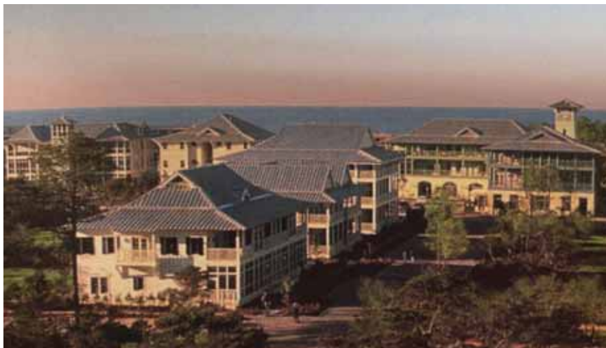
Many of WaterColor's multi-family units were roofed by SRD, Inc. of Birmingham, Ala., with Merchant & Evans' Zip-Rib in a mill-finish .032 aluminum.
