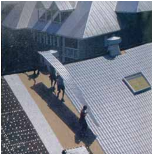
Metal, metal, everywhere. A crew from the Bob Hilson Co., based in Key Largo and Broward, carries a Berridge S-tile panel onto the roof of the historic Clinton Square Market in Key West. Under guidance from the city's Historic Architectural Review Commission, the company replaced the hundred-year-old galvanized tiles with Berridge's product, a 24-ga. G90 S-tile painted with a Kynar 500/Hylar 5000 coating in a "Prewathered Galvalume" color. The building in the background is the Key West Hilton, roofed in 5-v crimp.
