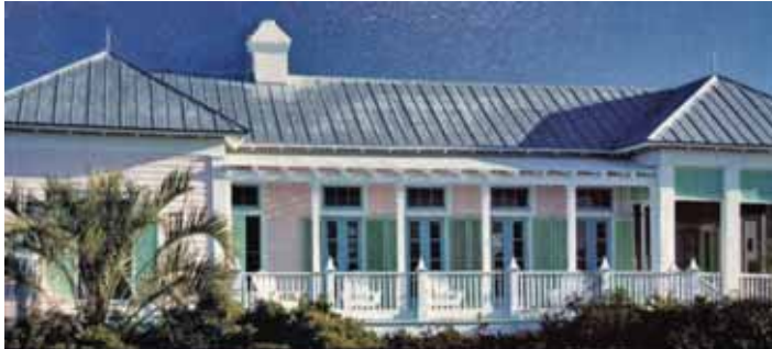
Seasiders don't insist on unblemished metal. The 5-v crimp roof on this Caribbean cottage, designed by Cooper Johnson Smith Architects, characterizes the casual, real-metal look preferred by many Floridians. But some newer Seaside homes are upgrading to more durable and corrosion-proof panels. (Photo: George Cott/Chroma)
