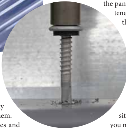
Take care to install screws perpendicular to the substrate.
