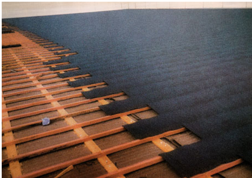
The Gerard Shake went on over a vast latticework of fire-proofed battens. (HORN BROS. PHOTO)
