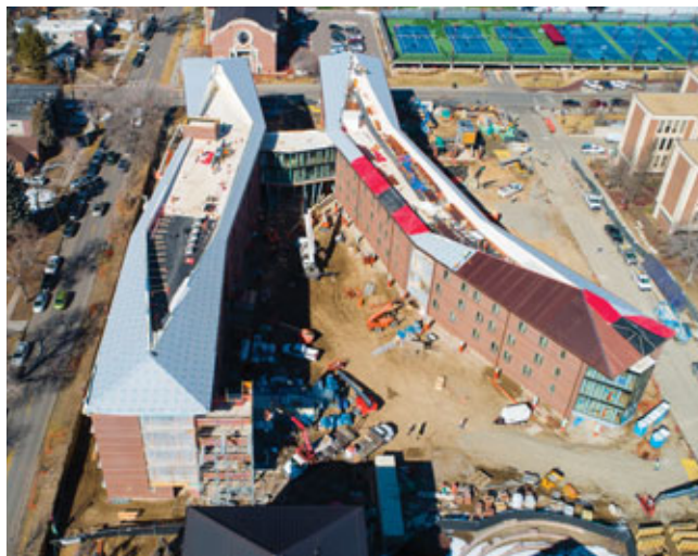
More than 30,000 sq. ft. of natural copper covers Denver University’s new Dimond Family Residential Village. Underlayment by Kirsch/Sharkskin. Photo courtesy of Schafer and Co., Denver, Colorado.
