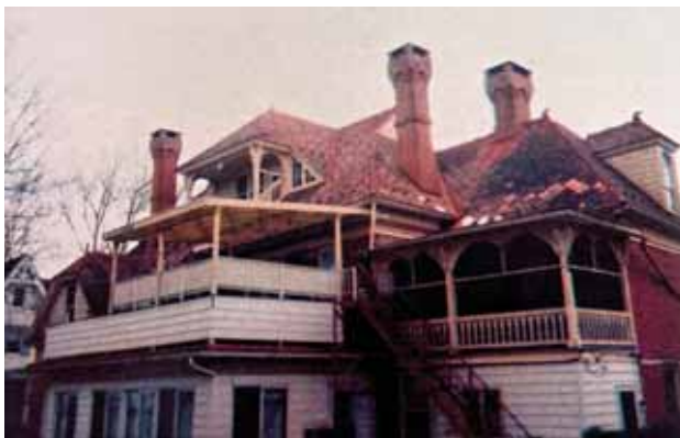
Crumbling, discolored, and leaking, this asbestos tile roof is history. (TREGO PHOTOS)
