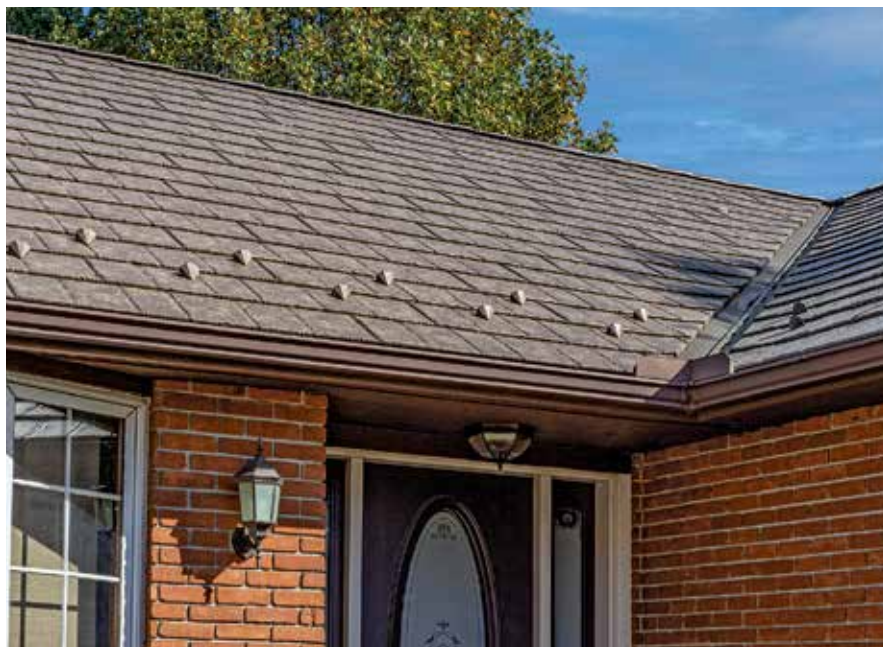
Residence roofed with ProVia Ironstone Slate metal shingle panels. Note the matching snow guards and their placement. PHOTO COURTESY PROVIA.
