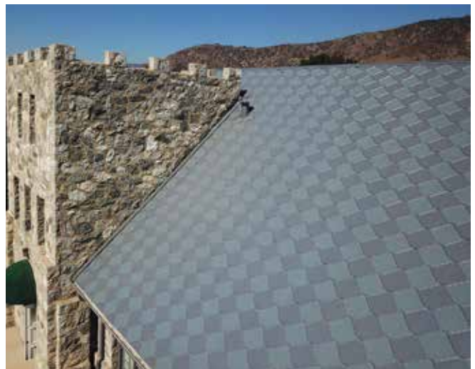
When the old asbestos diamond-shaped shingles began to fail on the Cornerstone Bible Church in Glendora, California, ATAS International's CastleTop diamond shingles were chosen as a replacement. (Recommended minimum slope of 3:12.) PHOTOS COURTESY OF ATAS INTERNATIONAL.
