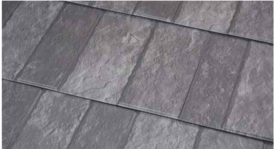
Courses are staggered, avoiding a direct repeat of likes in successive courses. Shown here is Milan Gray Slate from McElroy Metal. PHOTO COURTESY MCELROY METAL
