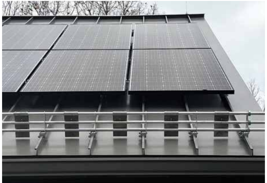
Allow space between the PV array and the eave so that snow can begin to slide off the panels before it contacts the snow rails. Plan ahead if solar will be added to a roof in snow country. PHOTO COURTESY ACECLAMP
