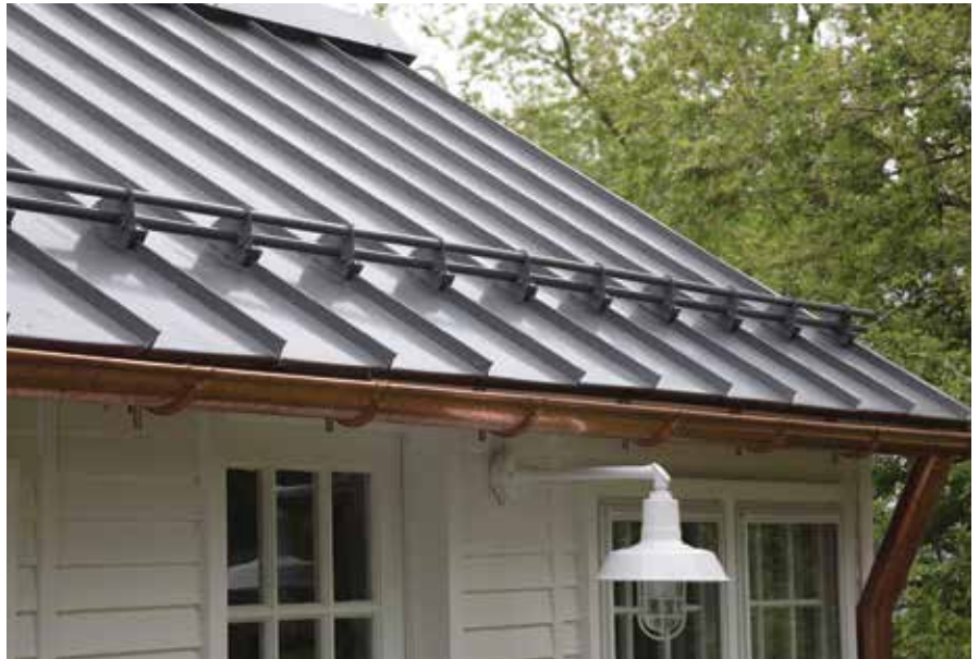
Snow rails are installed directly above a structural wall. PHOTO COURTESY ACECLAMP
