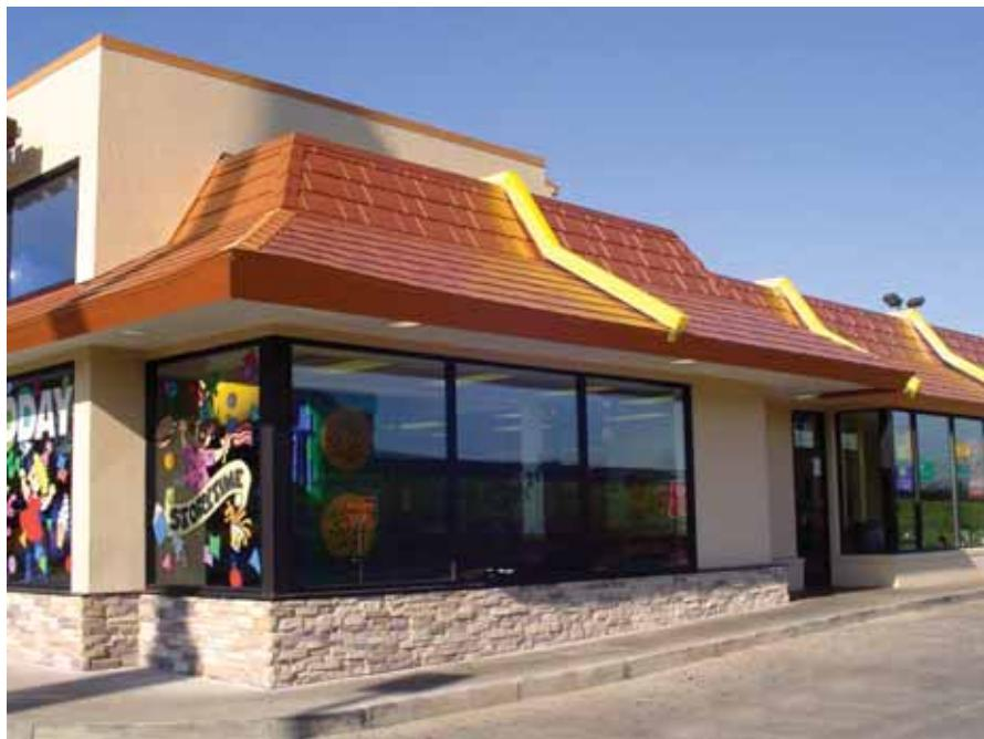
Premium cool coatings for metal substrates provide improved reflectivity, which helps reduce energy consumption.
