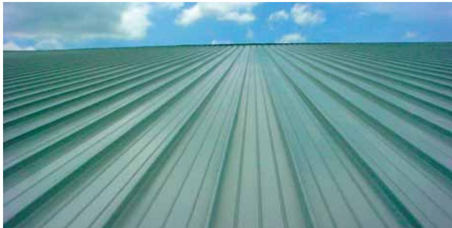
Standing seam metal roofs have simple, clean lines and can be finished in different styles and configurations.
