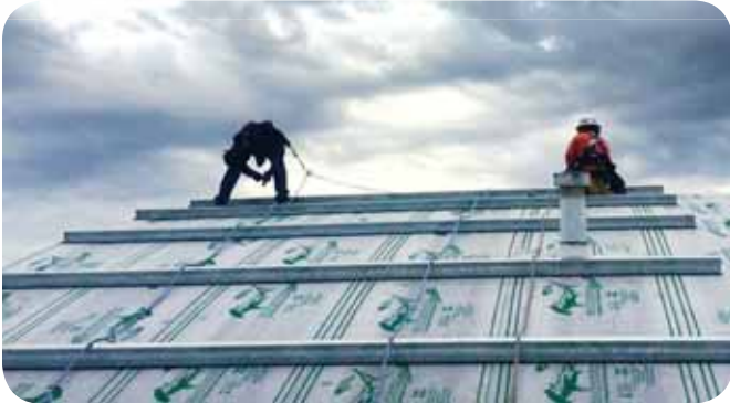
Photo courtesy of Tremco, Contractor Eberhart Roofing and Waterproofing, Jobsite Newbury Park, CA
