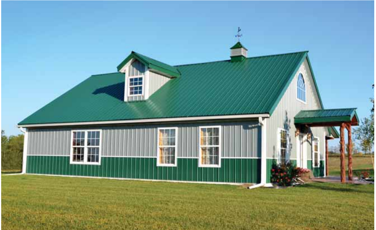
PHOTO COURTESY OF EVERLAST ROOFING
