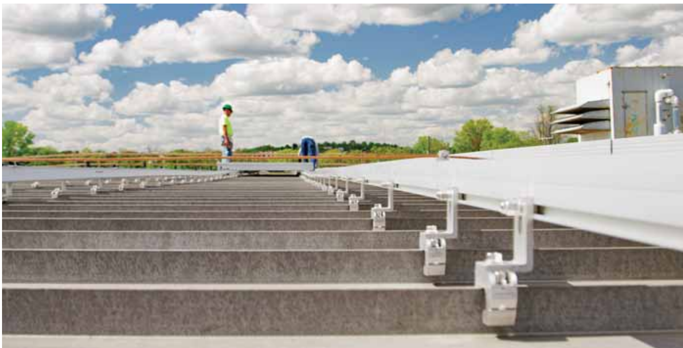
Systems installed on low-sloped metal roofs may be more affected by high snow loads. Be sure to follow the local codes for wind uplift and snow loading for whatever the roof slope is.
