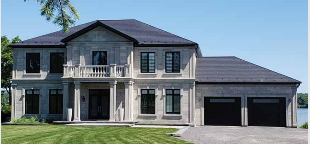
PHOTO COURTESY OF IDEAL ROOFING
