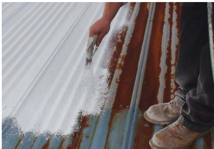
Coatings can be applied to older (even rusted) roofing panels if the necessary preparation steps are completed. Photo courtesy of Ames Research Laboratories.
