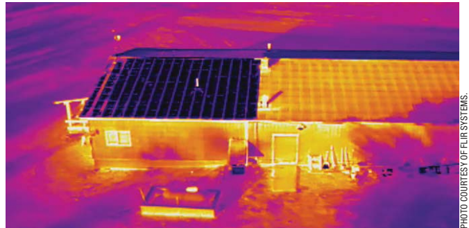
PHOTO COURTESY OF FLIR SYSTEMS.
