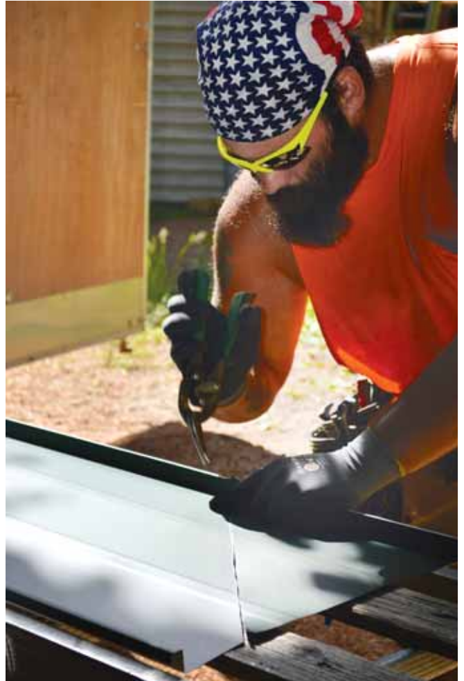
Crew member Dave Lancour uses snips to create a custom cut.
