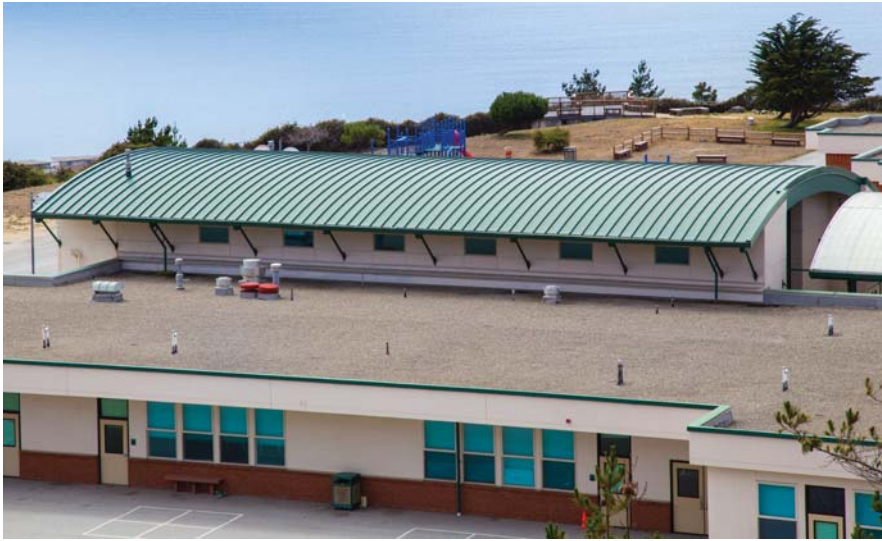
Elementary school on the West Coast featuring a curved metal roof—note the proximity to the shoreline. Photo courtesy of The Garland Company.
