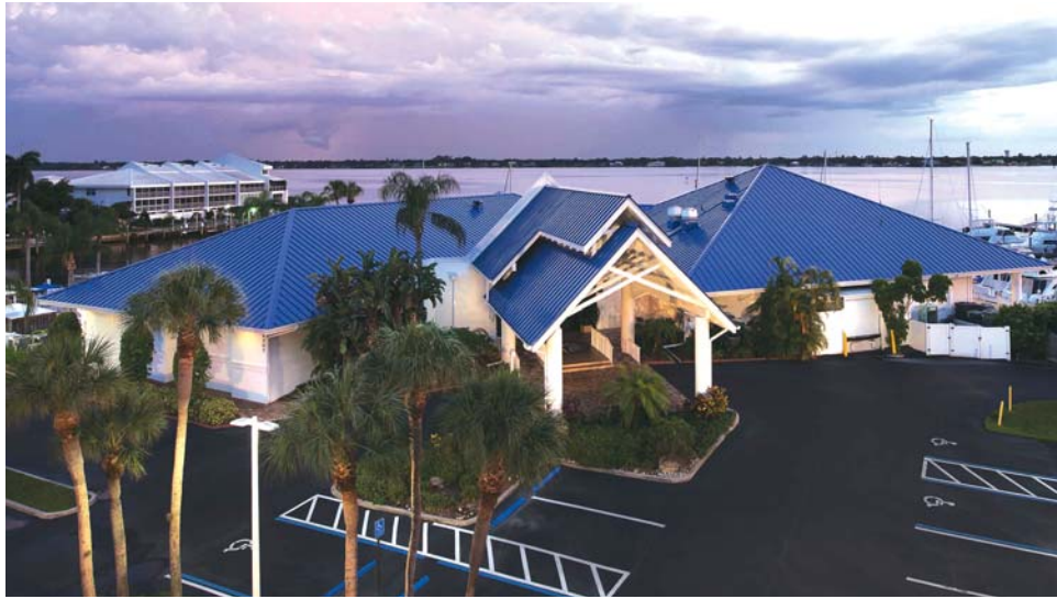
The new blue aluminum roof on the Bradenton Yacht Club in Bradenton, Florida, replaced an old, tired roof, giving the building new life. Photo courtesy of PAC-CLAD and www.hortonphotoinc.com .
