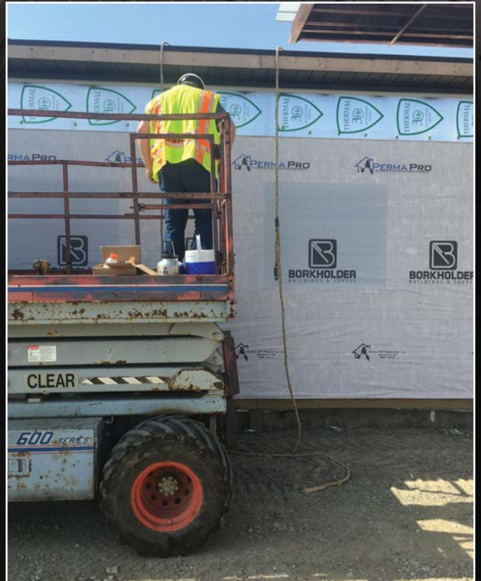
An OSHA inspector measures potential fall distance based on the actual rope being used. This real, un-staged inspection resulted in a fairly hefty fine.
