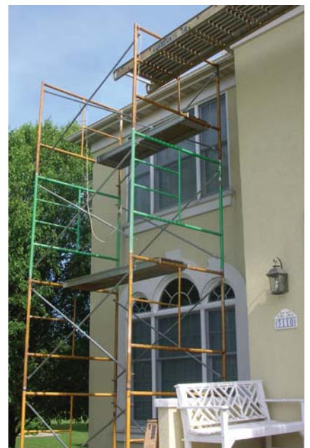
If using scaffolding, it must meet strict standards for safety.
