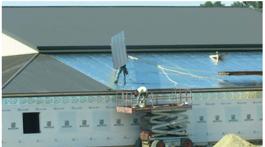
Photos taken from a distance by an OSHA inspector, prior to speaking with the job site manager. All images provided by Todd Meinhold.
