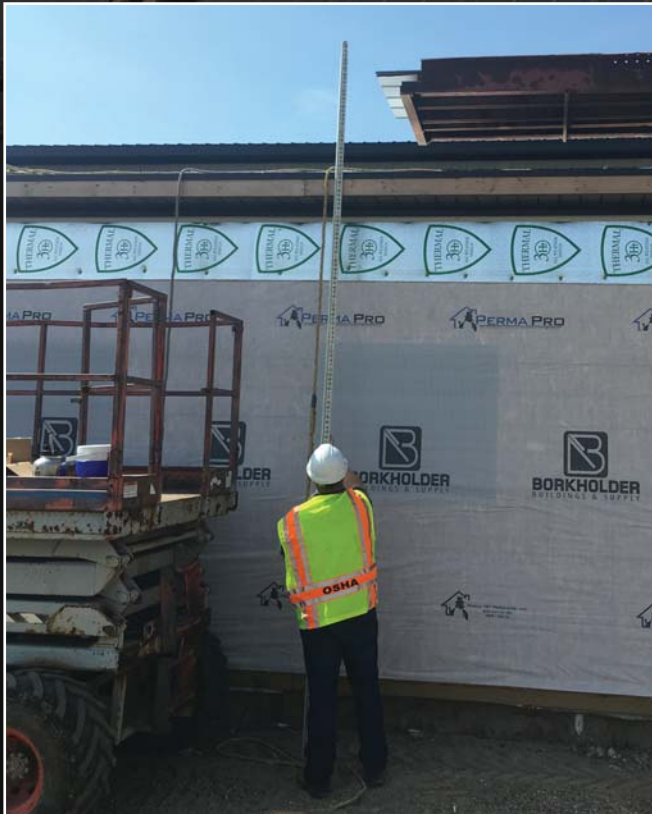
An OSHA inspector measures potential fall distance based on the actual rope being used. This real, un-staged inspection resulted in a fairly hefty fine.
