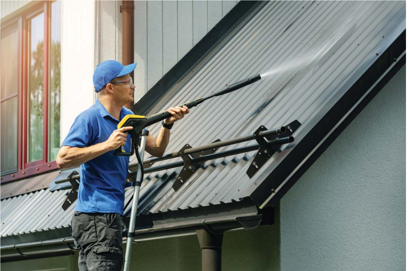
High-pressure power washers run the risk of damaging the coating on a metal roof, which in turn can void the warranty. Always consult the panel and coating manufacturer for their recommendations on panel cleaning and maintenance.
